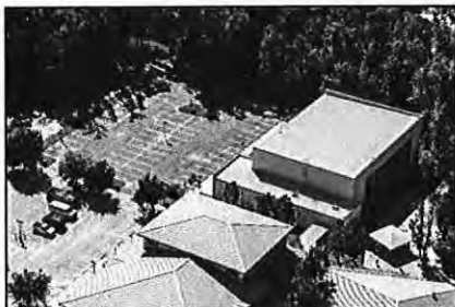
Building & Parking Aerial
