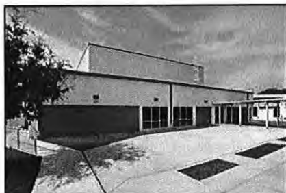
Main Entrance with Covered Walkway
