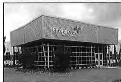
LEED GOLD EnviroFocus Hygiene & Office Building
