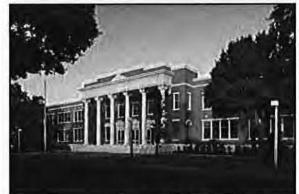
Completed Project Photograph
