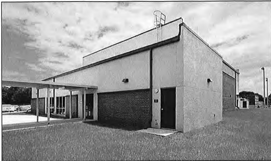
New Building Façade
