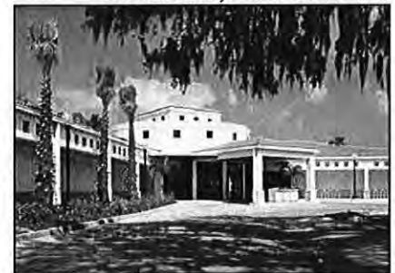
Safety Harbor Public Library Expansion
