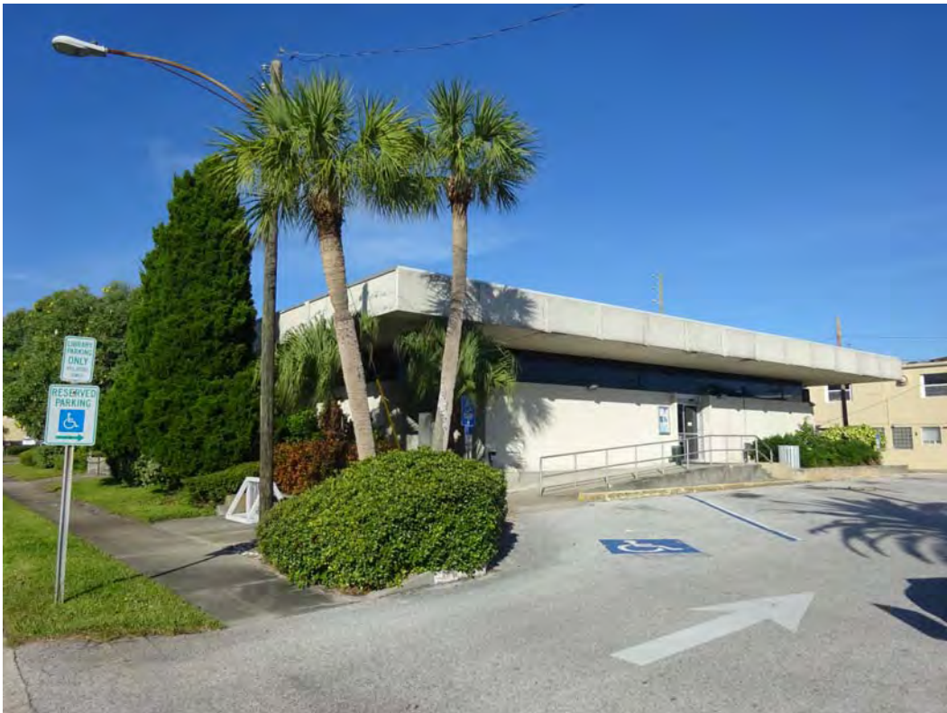
General views of the building exterior
