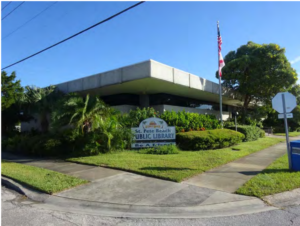
General views of the building exterior
