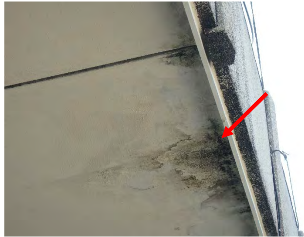
Picture 11 – Example of Roof Soffit
