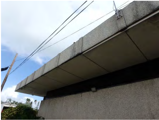
Picture 10 – Example of Roof Fascia Panels
