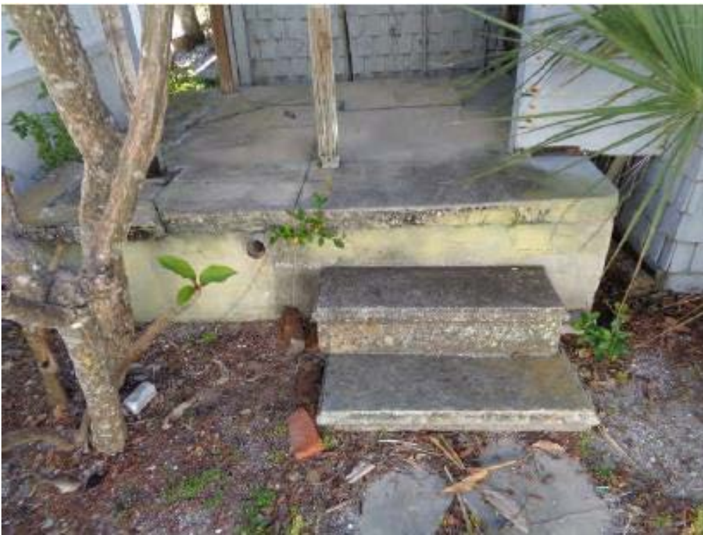
Figure 8 - Cistern at rear of the cottage
