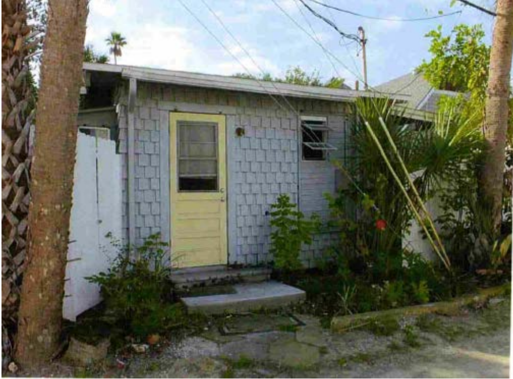
Figure 7 - Rear (north side) of the cottage, 113 10 th Avenue
