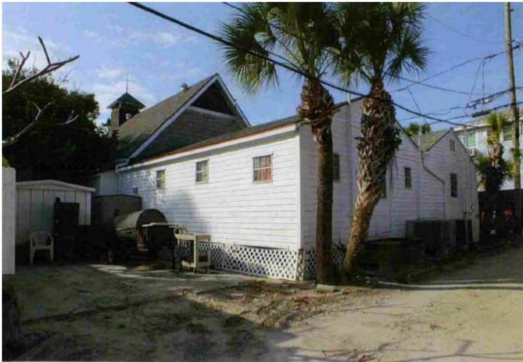
Figure 4 - Rear addition (former army barracks), 115 10th Avenue
