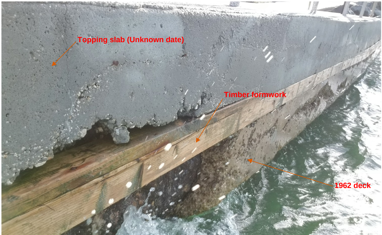
Figure 2-6 Deck Elevation – South Side
