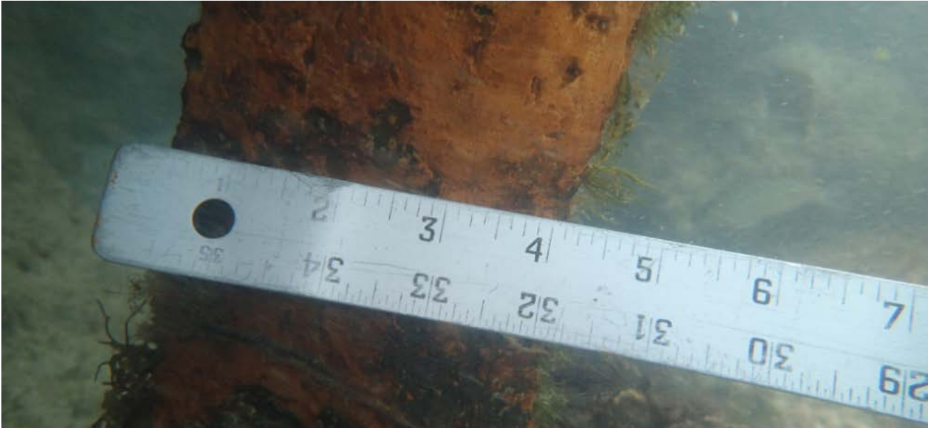
Figure 2-9 Typical Flange Condition
