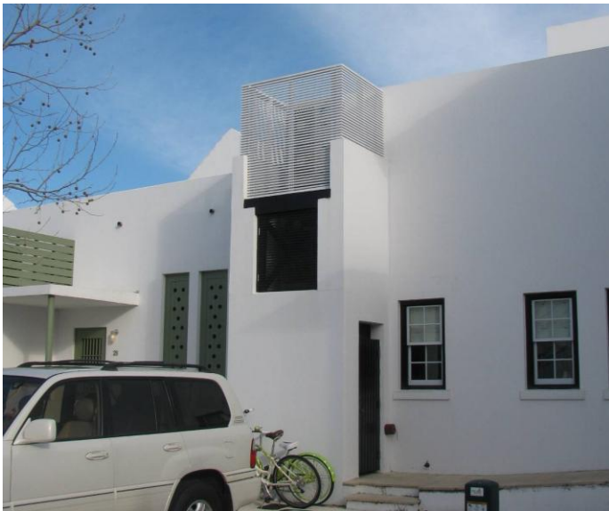
Conceal mechanical equipment from plain view wherever possible.
