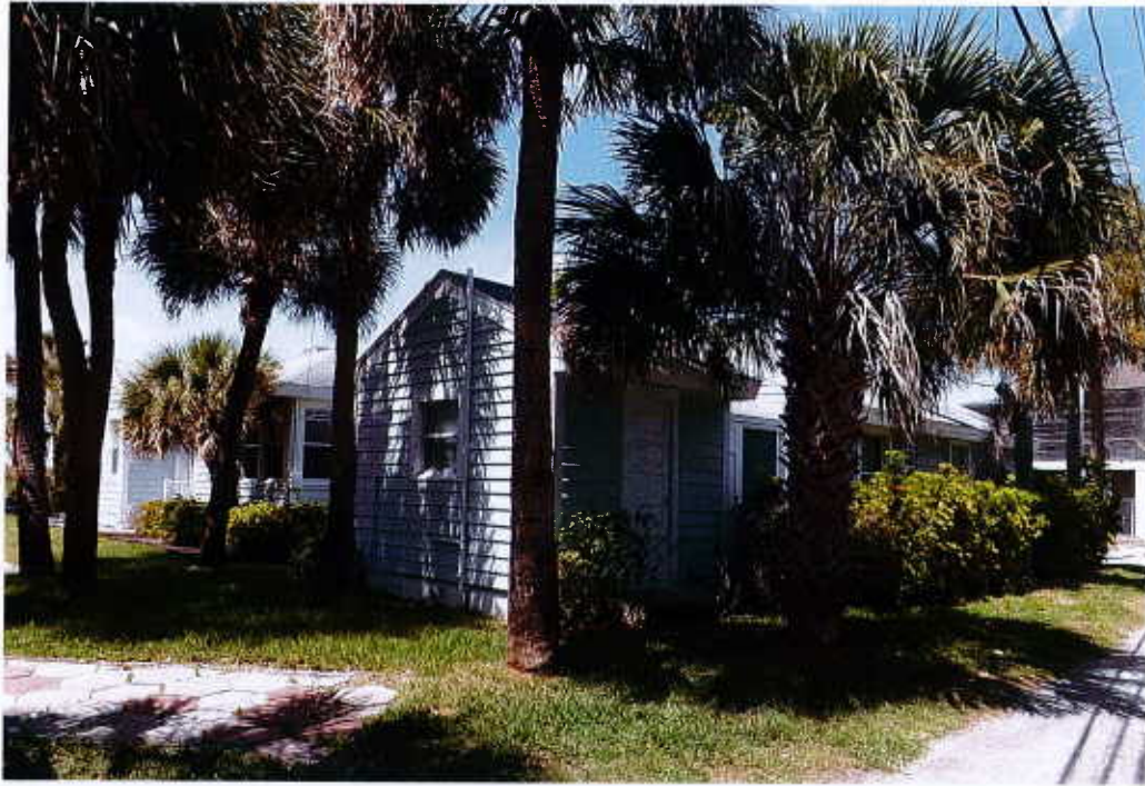
Figure 3 – Sunset Way toward rear of property
