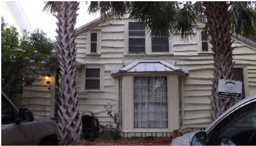
Exhibit A. Front of Structure
