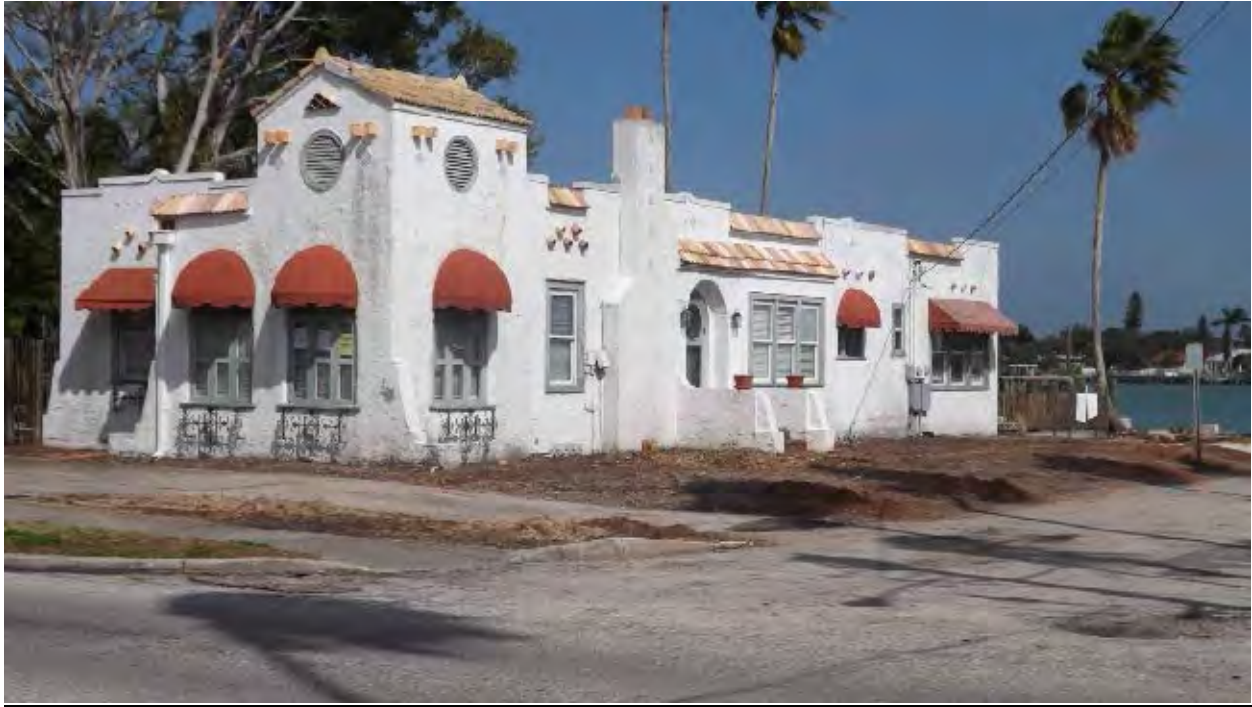
Exhibit B. View from slightly south on Pass-a-Grille Way
