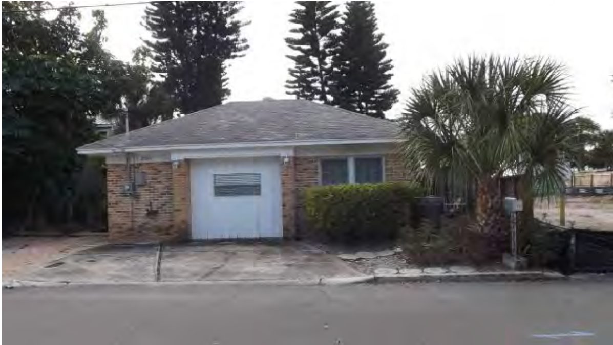
Exhibit A. View from Sunset Way (accessory structure)
