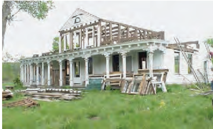
Dismantling of Bruchmann residence, May 2000
