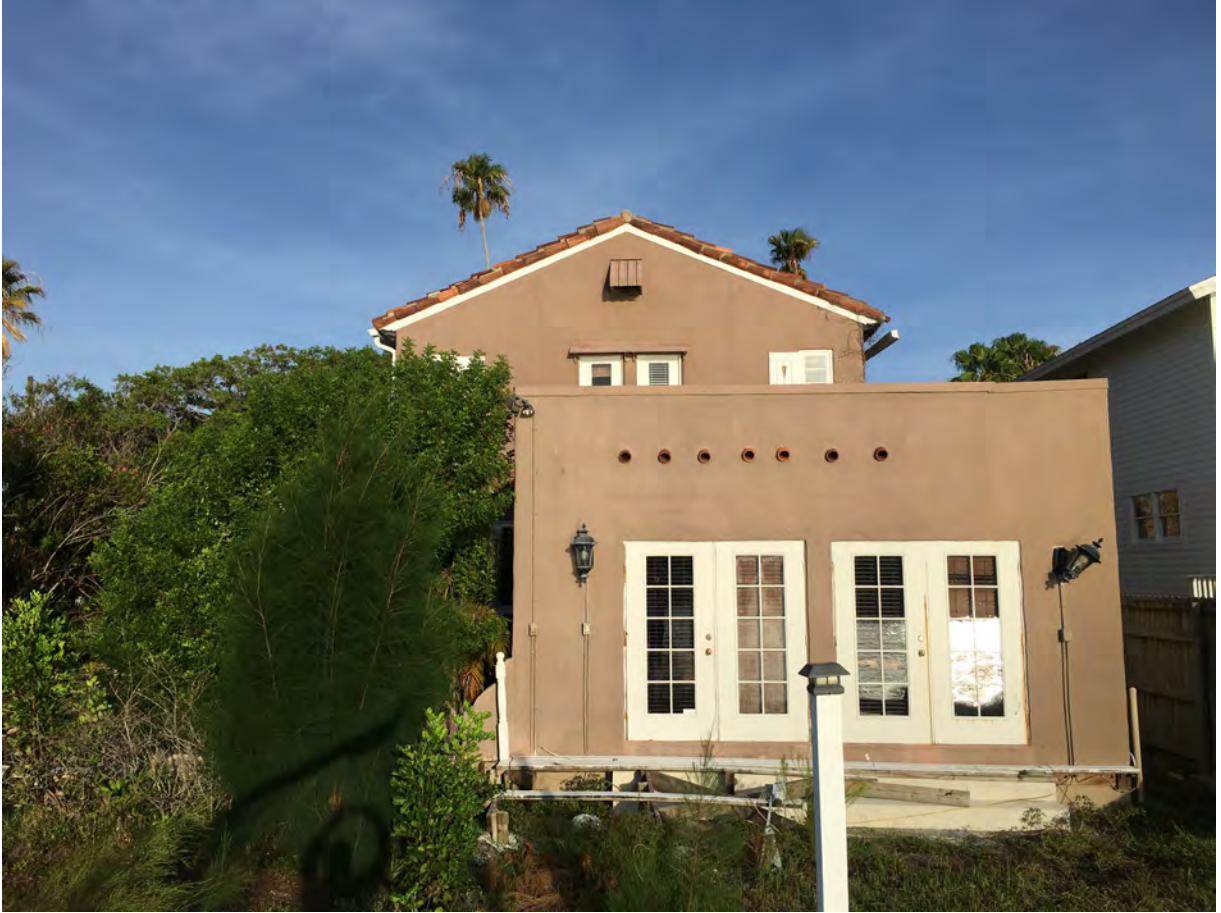
Subject Property Rear Elevation
