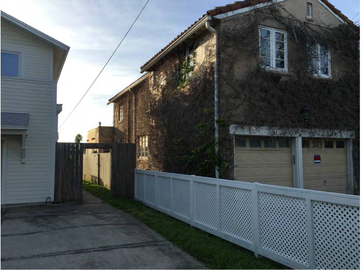
Subject Property Side (North) Elevation
