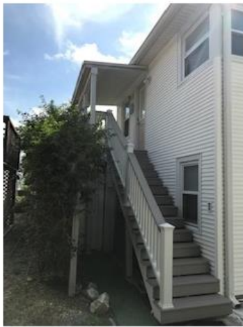
East elevation of GARAGE
