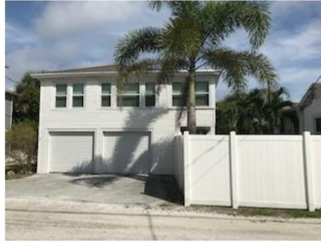
West elevation of GARAGE
