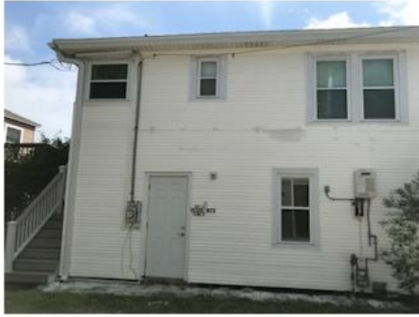
North elevation of GARAGE
