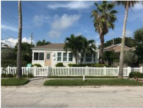
South Elevation of HOUSE
