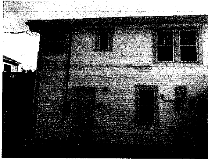
North elevation of GARAGE
