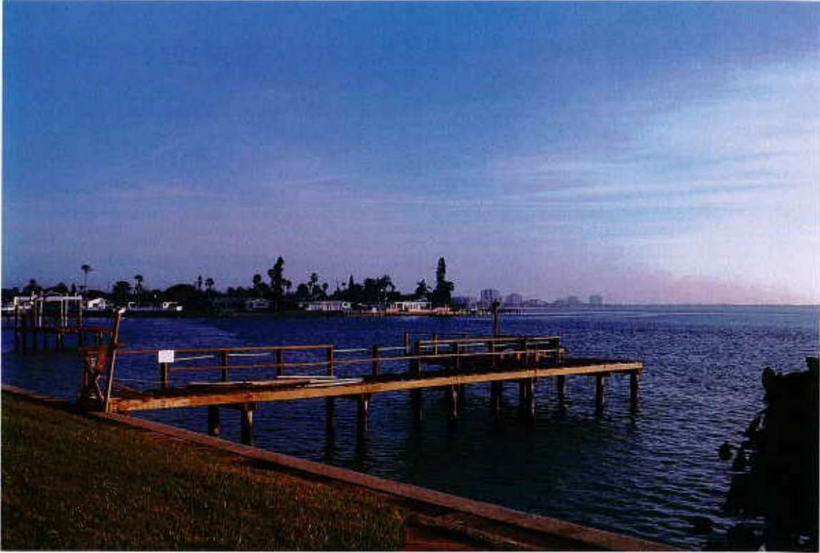
Figure 2. Storm Damaged Dock at 1505 Pass-A-Grille Way
