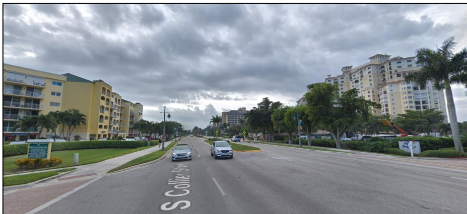
Collier Ave, looking south from Maple Ave
