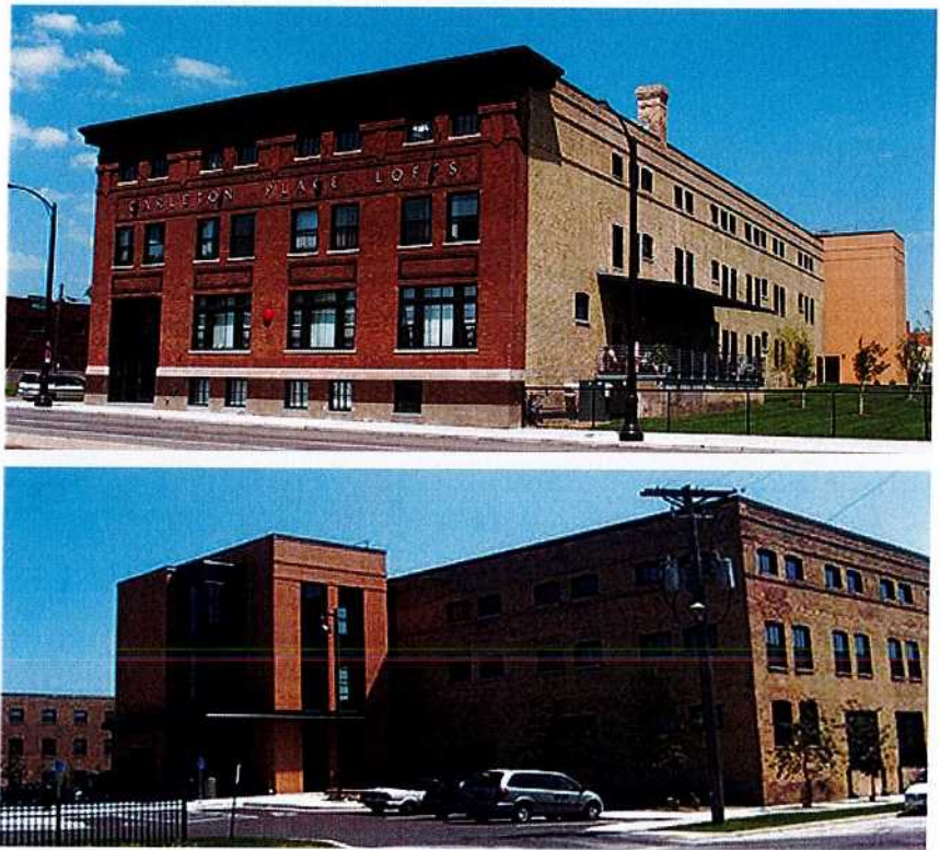
Figure 8. The rehabilitation of this large, early-20th century warehouse (top) into affordable artists' lofts included the addition of a compatible glass and brick elevator/stair tower at the back (bottom).
