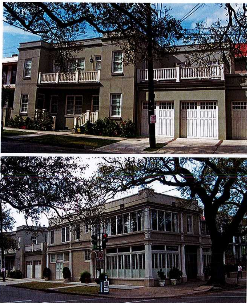
Figure 6. A new addition (top) is connected to the garage which separates it from the main block of the c. 1910 former florist shop (bottom). The addition is traditional in style, yet sufficiently restrained in design to distinguish it from the historic building.
