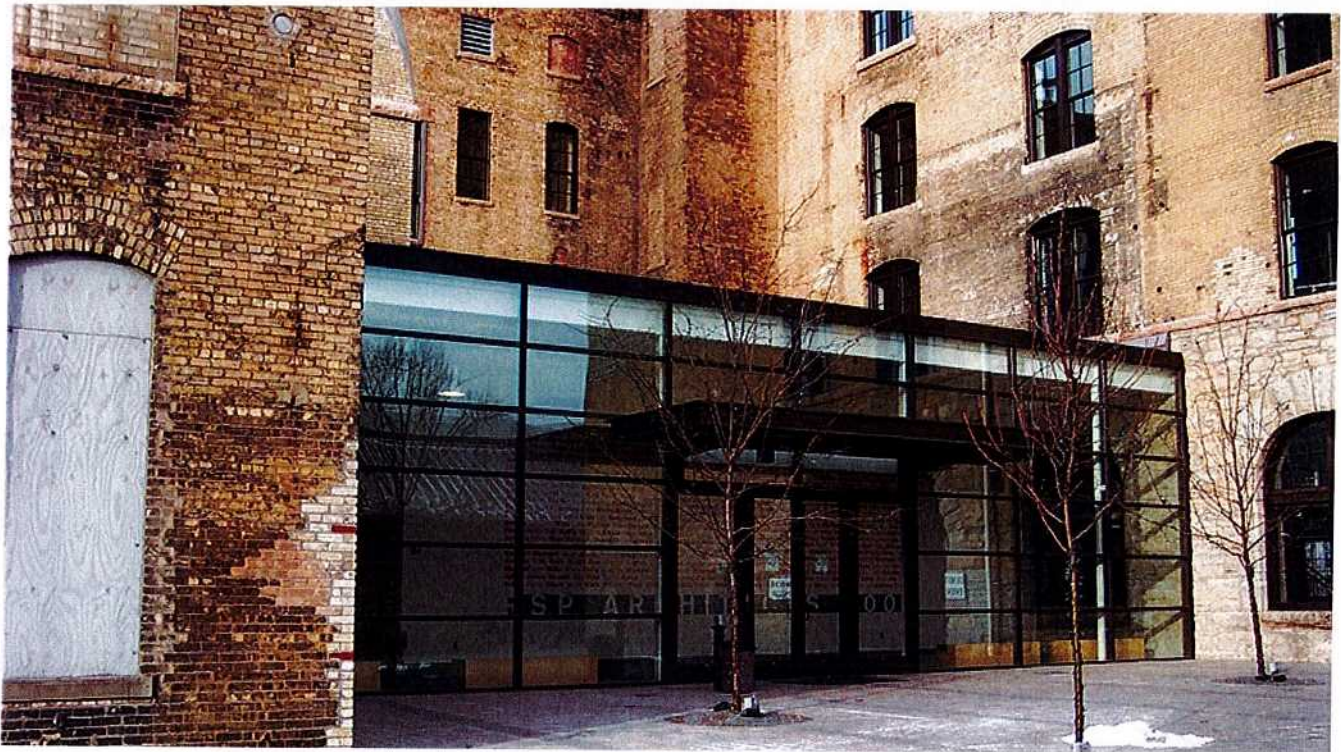
Figure 14. This glass addition was erected at the back of an 1895 former brewery during rehabilitation to provide another entrance. The addition is compatible with the plain character of this secondary elevation.
