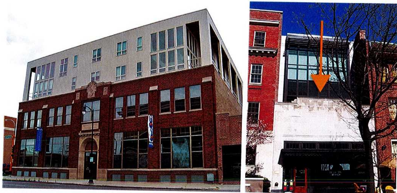
Figure 20. The height, as well as the design, of these two-story rooftop additions overwhelms the two-story and the one-story, low-rise historic buildings.
