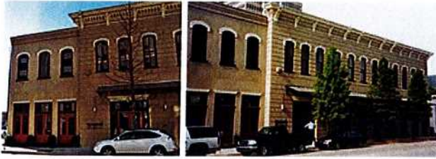
Figure 28. A small addition (left) was constructed when this 1880s train station was converted for office use. The paired doors with transoms and arched windows on the compatible addition reflect, but do not replicate, the historic building (right).
