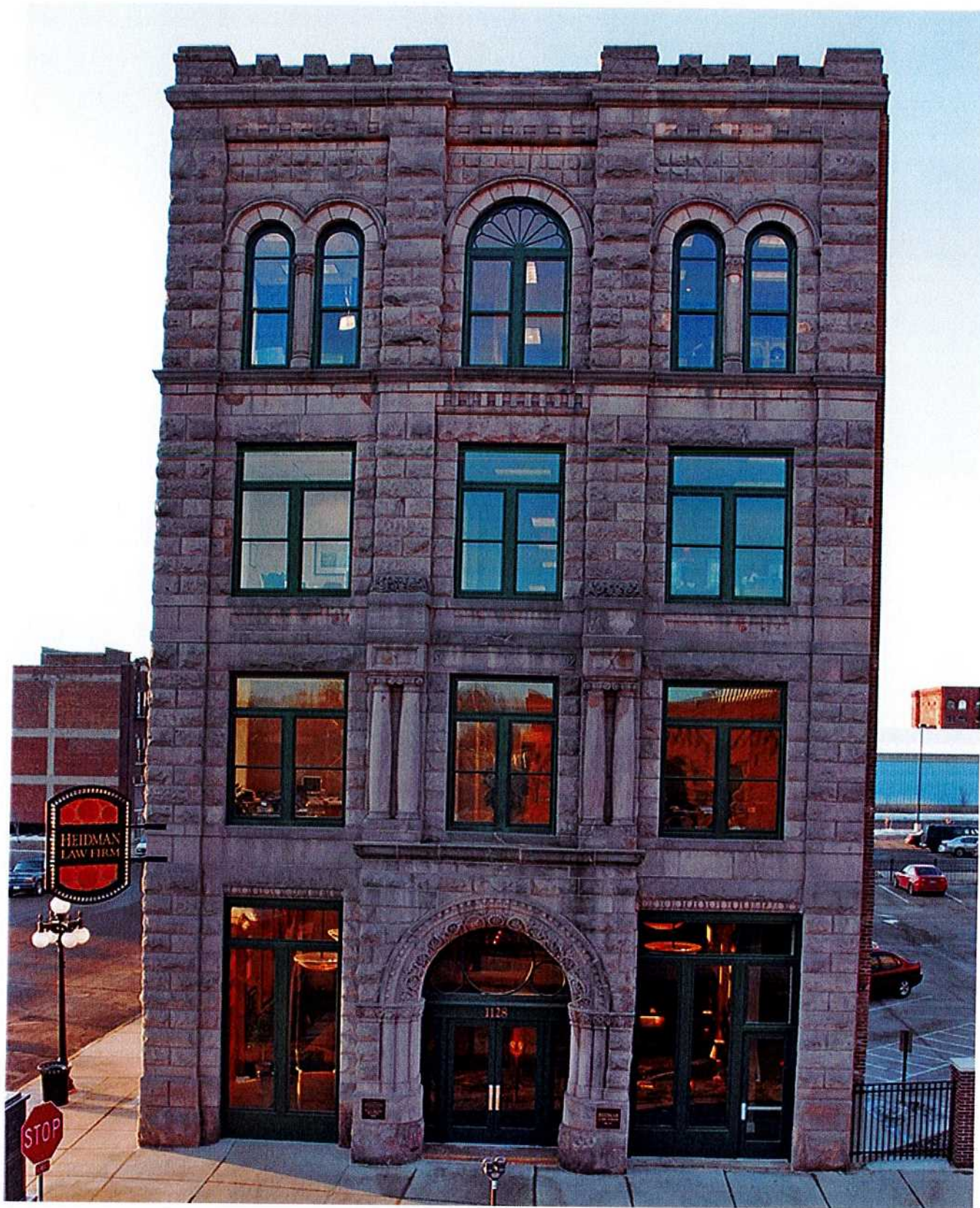
Figure 27b. Although the new brick stair/elevator tower (27a) is not visible from the front (27b), it is on a prominent side elevation of this 1890 stone bank. The compatible addition is set back and does not compete with the historic building. Photos: Chadd Gossmann, Aurora Photography, LLC.
