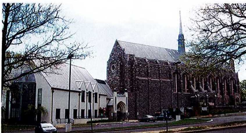
Figure 10. The small size and the use of matching materials ensures that the new addition on the left is compatible with the historic Romanesque Revival-style building.
