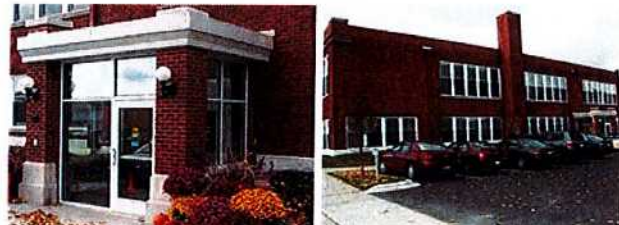
Figure 29. This simple glass and brick entrance (left) added to a secondary elevation of a 1920s school building (right) is compatible with the original structure.
