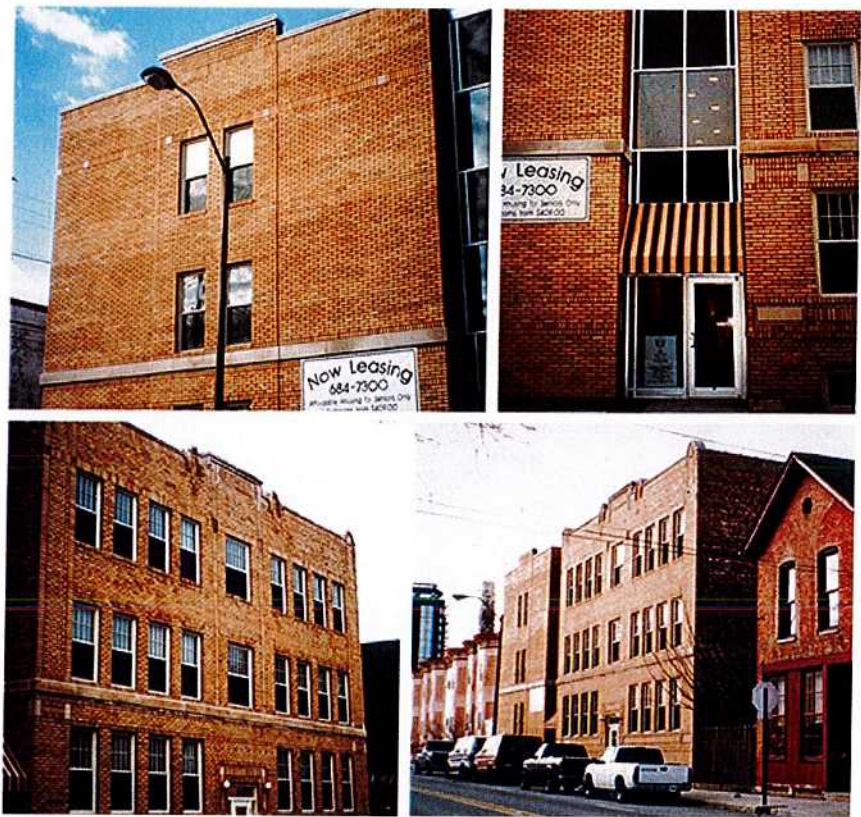
Figure 5. This addition (top left) is constructed of matching brick and attached by a recessed connector (top right) to the 1914 apartment building (bottom left). The design is compatible and the addition is smaller and subordinate to the historic building (bottom right).
