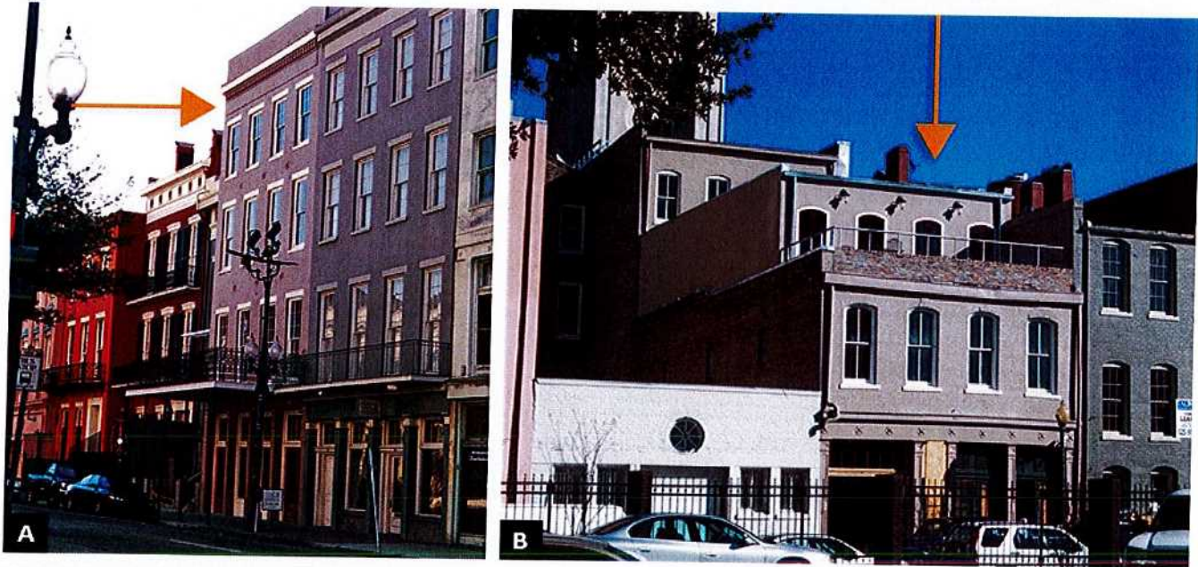
Figure 26. (A) A rooftop addition would have negatively impacted the character of the primary facade of this mid-19th century, four-story structure and the low-rise historic district. (B) A third floor was successfully added on the two-story rear portion of the same building with little impact to the building or the district because it blends in with the height of the adjacent building.
