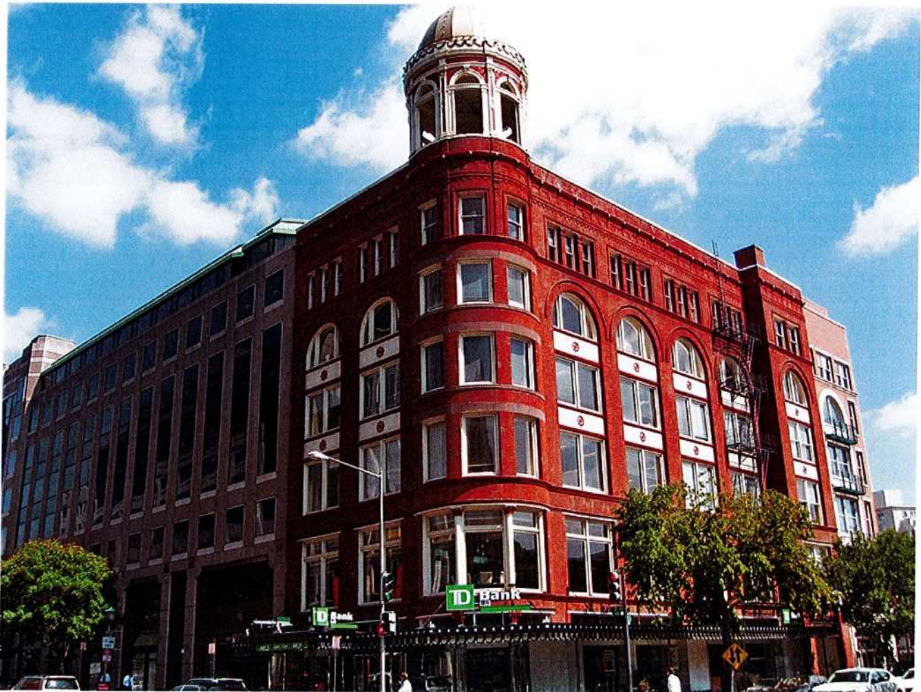
Figure 30. The small addition on the right of this late-19th century commercial structure is clearly secondary and compatible in size, materials and design with the historic building.
