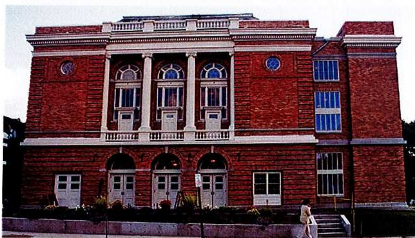
Figure 7. A vacant side lot was the only place a stair tower could be built when this 1903 theater was rehabilitated as a performing arts center. Constructed with matching materials, the stair tower is set back with a recessed connector and, despite its prominent location, it is clearly subordinate and differentiated from the historic theater.
