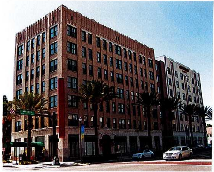
Figure 2. The new section on the right is appropriately scaled and reflects the design of the historic Art Deco-style hotel. The apparent separation created by the recessed connector also enables the addition to be viewed as an individual building.
