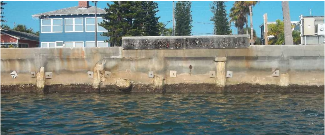
Figure 3-9 Tiebacks Between Stations 5+00 and 6+00
