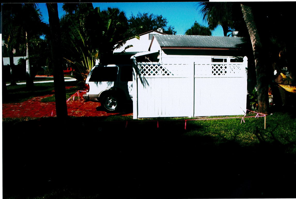
LOOKING NORTHWEST NOTE PINK RIBBON OUT LINEING GARAGE
