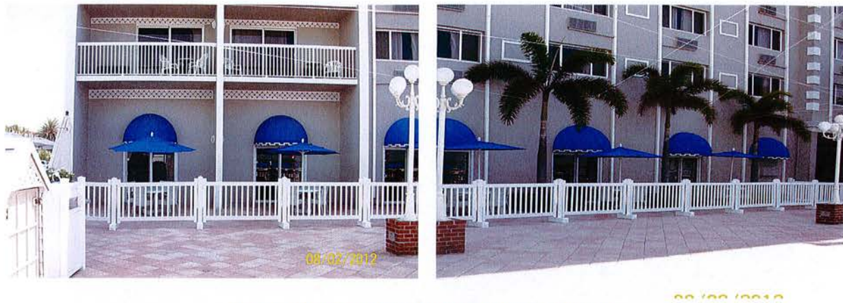
Figure 1 - View Toward Hotel and Front Canopy Location
