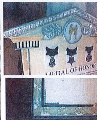
Molds were pulled from existing elements in the Capitol to match border and original Kentucky Seal
