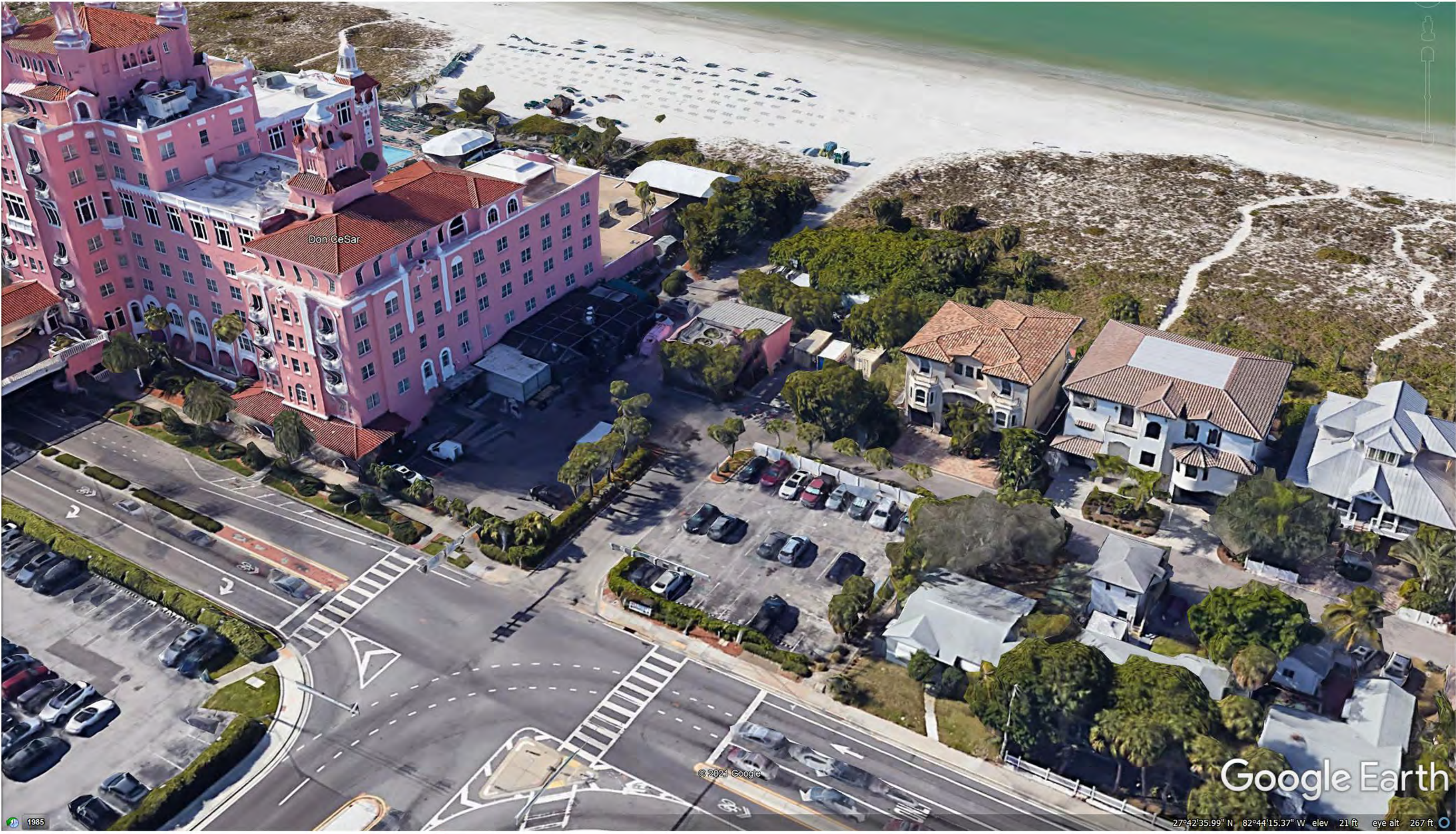
1 EXISTING AERIAL VIEW OVER GULF BOULEVARD A3.1 NTS
