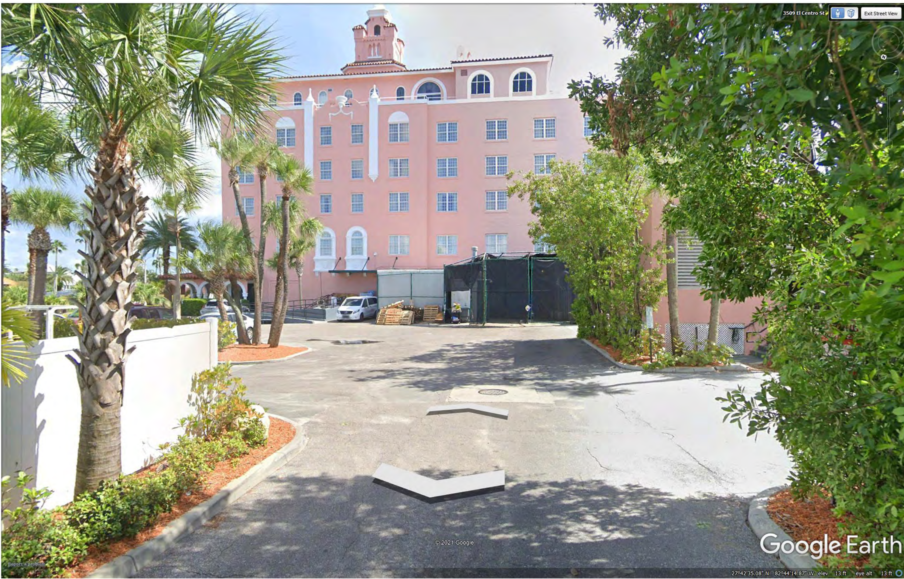
2 EXISTING VIEW FROM EL CENTRO STREET A3.1 NTS
