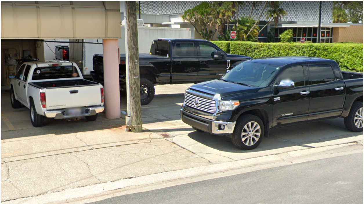
Concrete curb and apron deterioration at Fire Station 23 along 73 rd Avenue.
