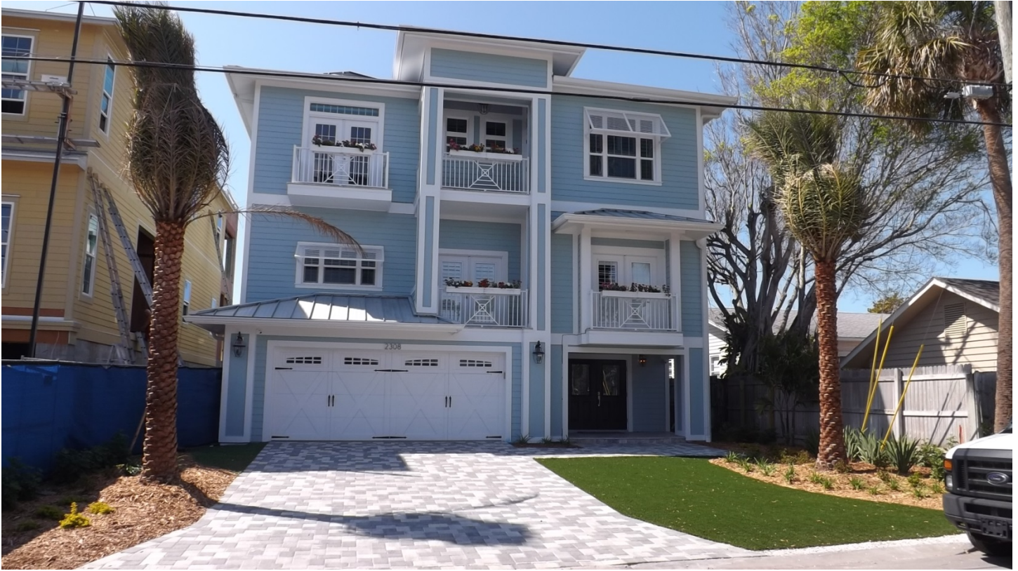
Above: Subject property facing west, current conditions
