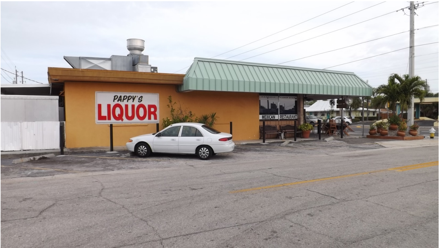
Above: Subject property, viewed from 64 th Avenue facing north
