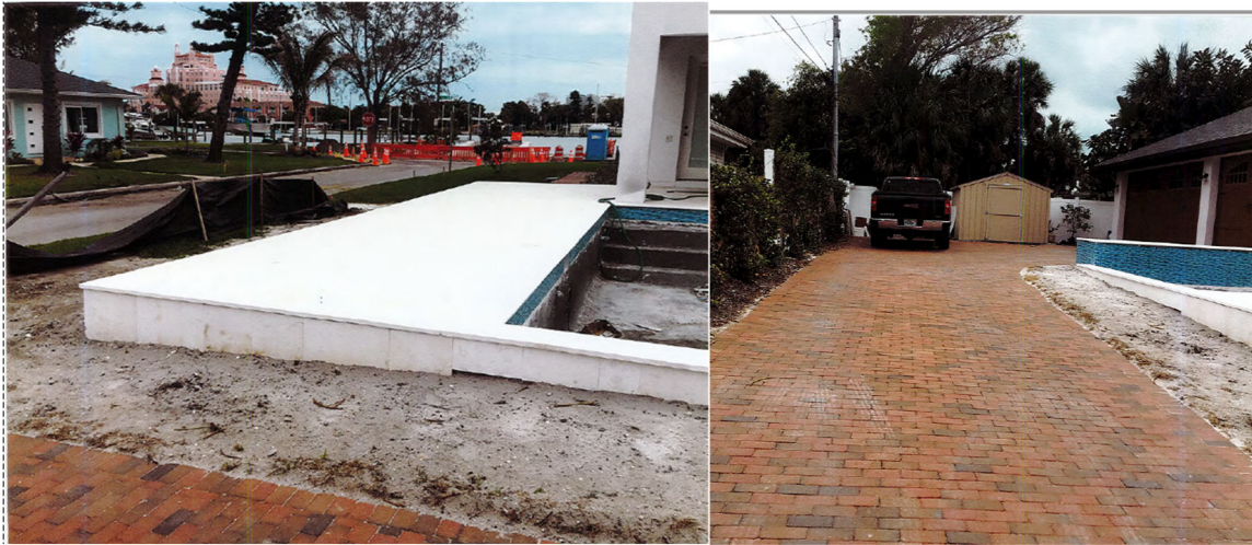
Pool area under construction (top left and right). Pool Deck 17-inch above grade.
