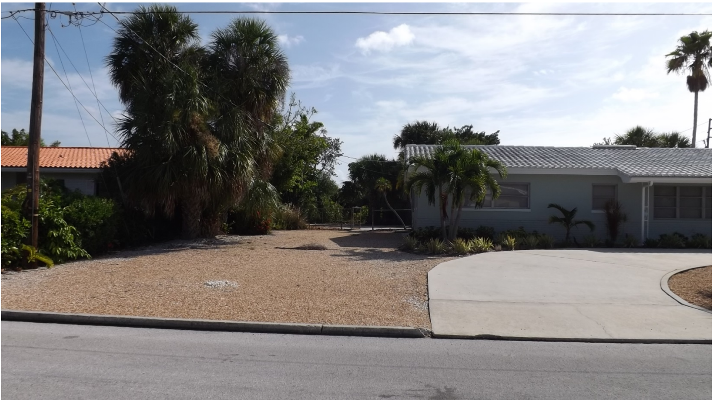
Above: Area of proposed construction, facing northeast.
