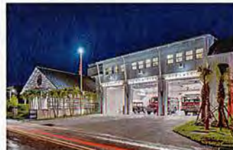
CAPTIVA ISLAND FIRE STATION CAPTIVA, FL
