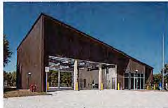
BRIGHTON FORESTRY FIRE STATION, BRIGHTON, FL
