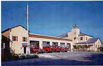
BOCA GRANDE FIRE DEPARTMENT BOCA GRANDE, FL
