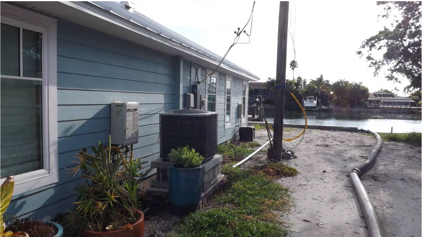
Above: Subject property, facing east; proposed pool equipment location
