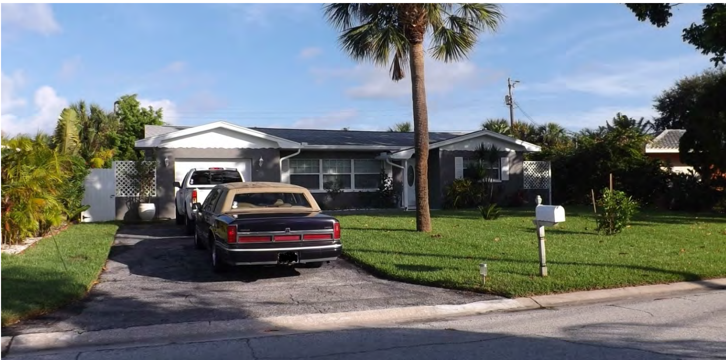
Above: Subject property, facing north
