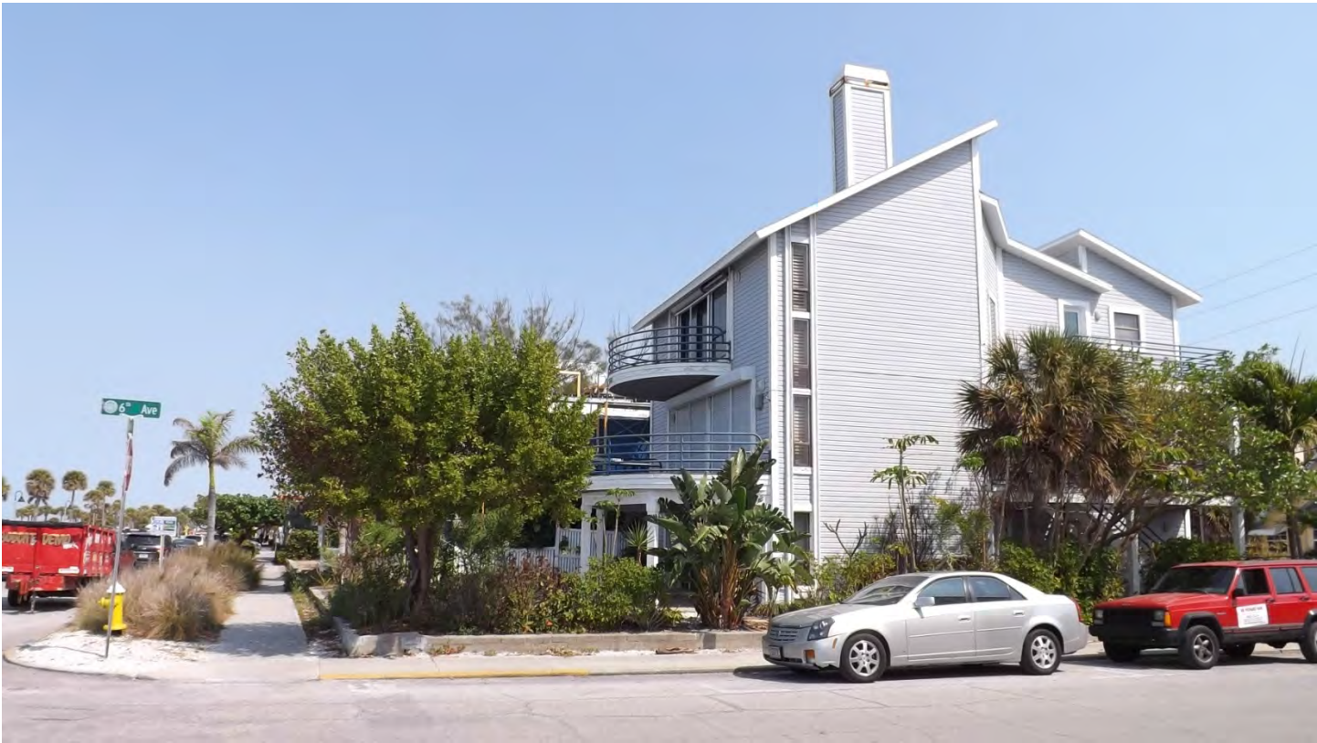
Above: Subject property, facing north
