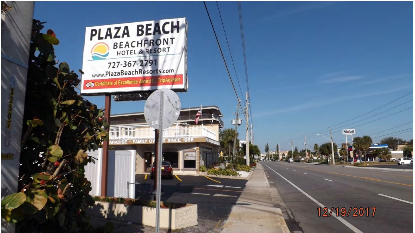
Above: Subject property, facing north
