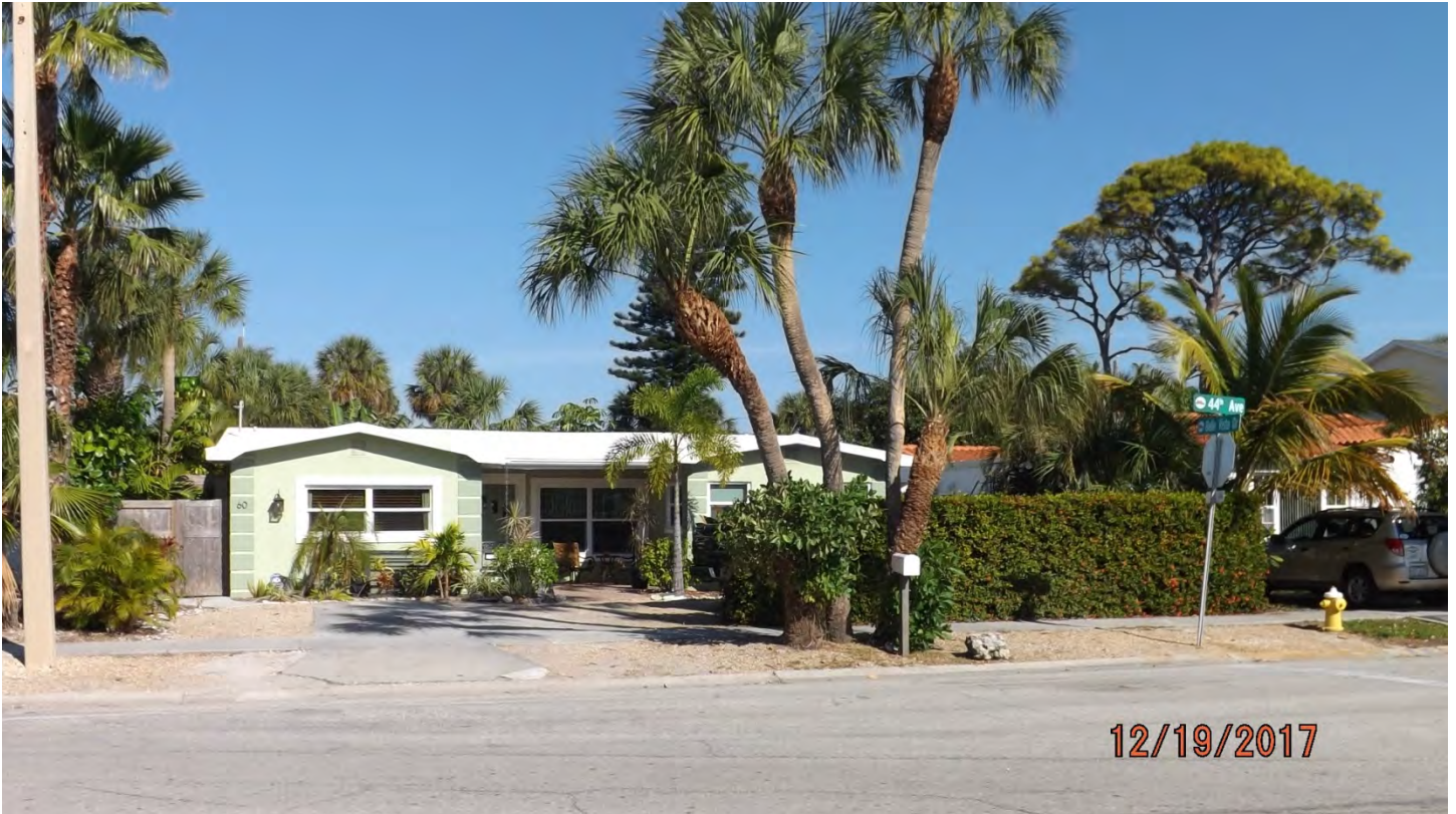
Above: Subject property, facing north
