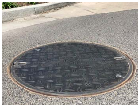
Composite cover shown in an iron frame.
