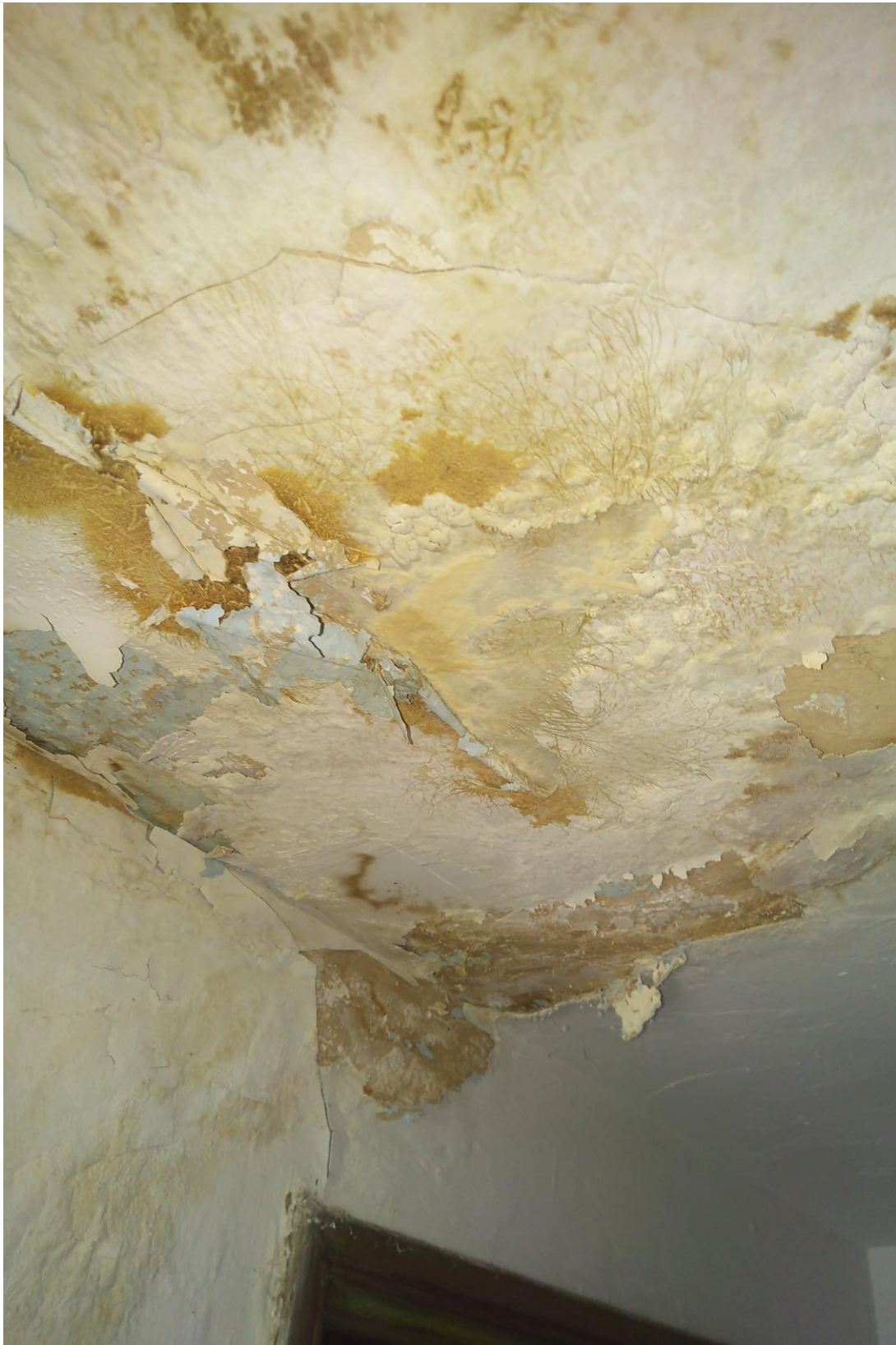
Collapsing Plaster
