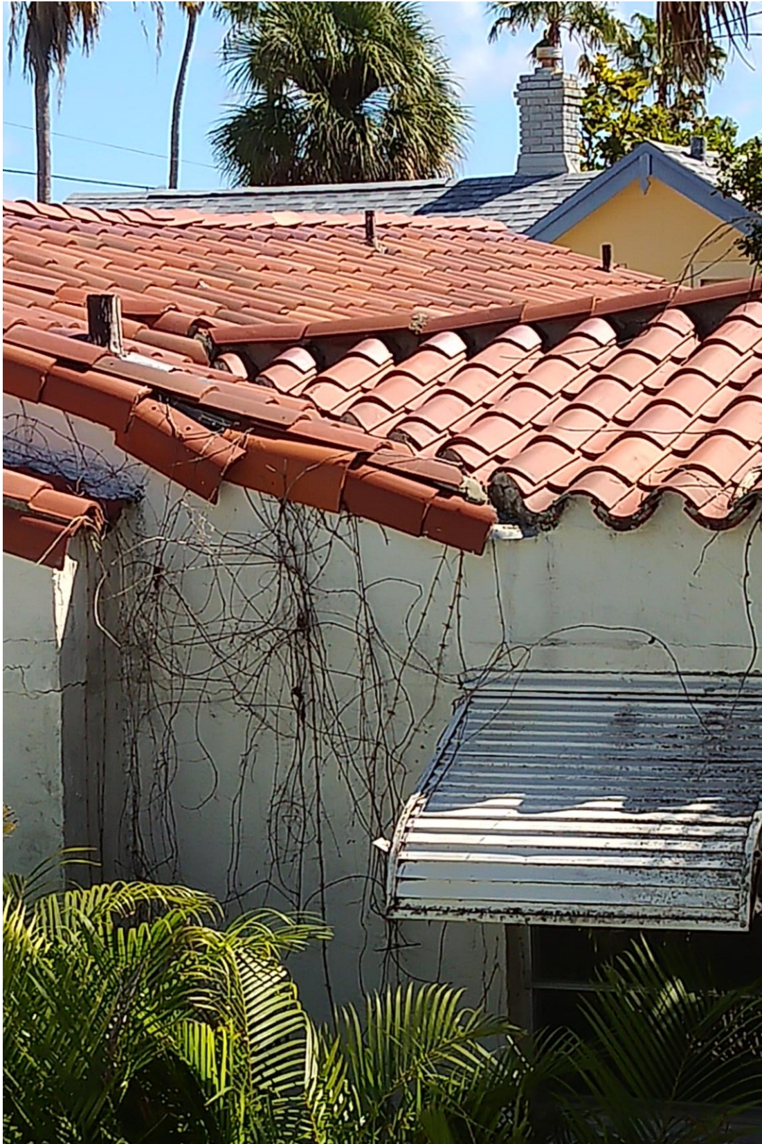
Failing Roof
