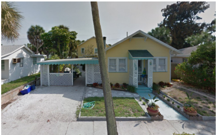
Figure 3: Home featuring carport addition
