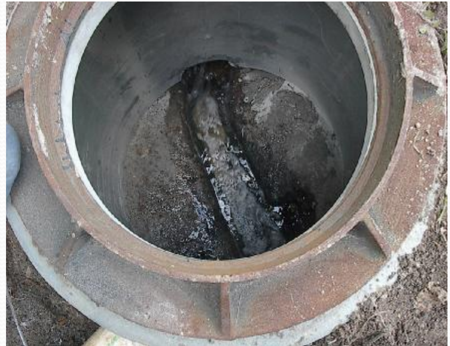
Repair with Fiberglass Liners
