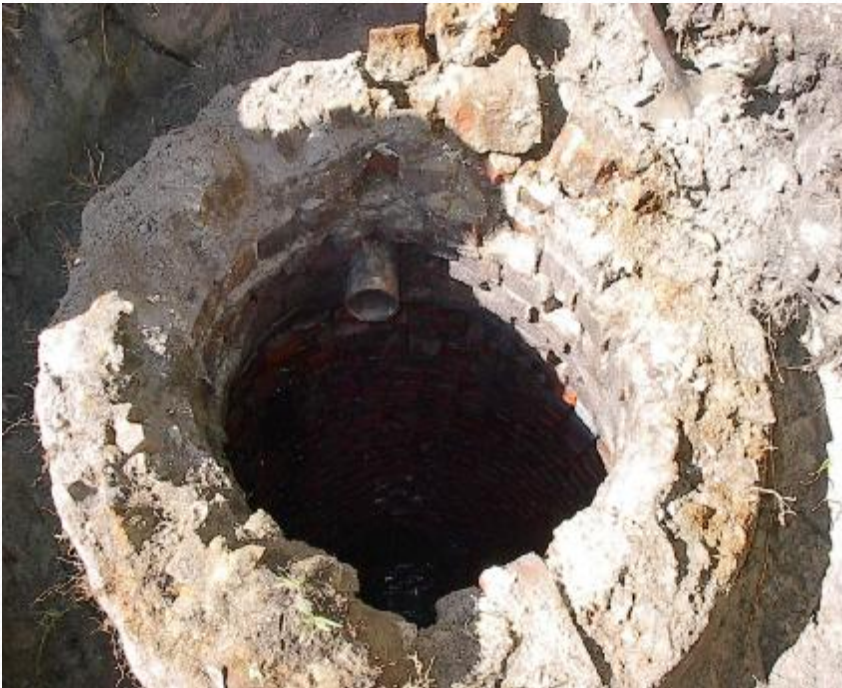
Deteriorating Manholes
