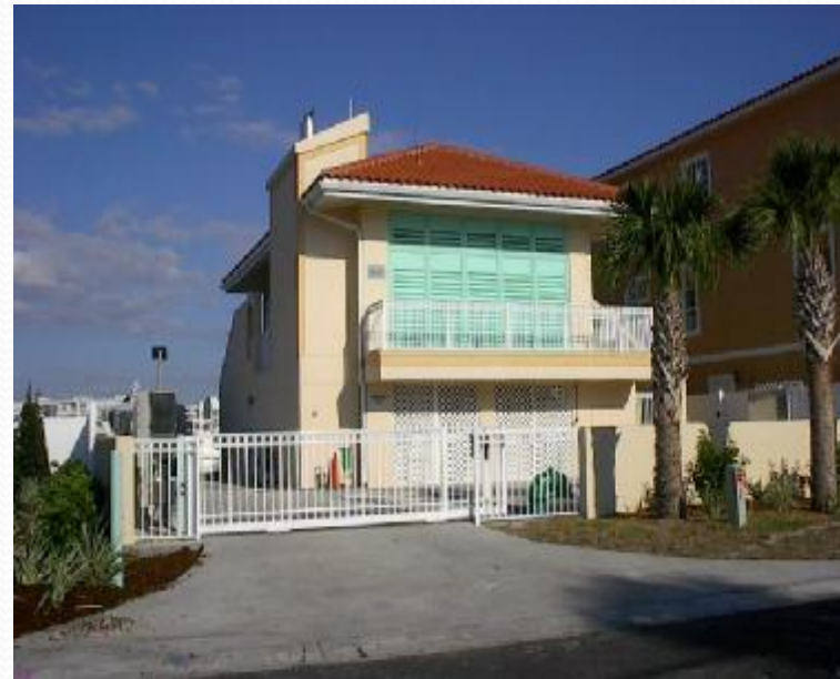
New Master Pump Station
