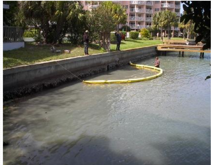
Spill Containment at Outfall
