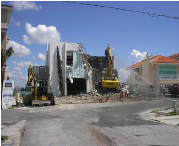
Old Pump Station
