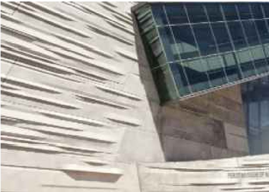
PC-01 PRECAST CONCRETE PANEL - TYPE 1
