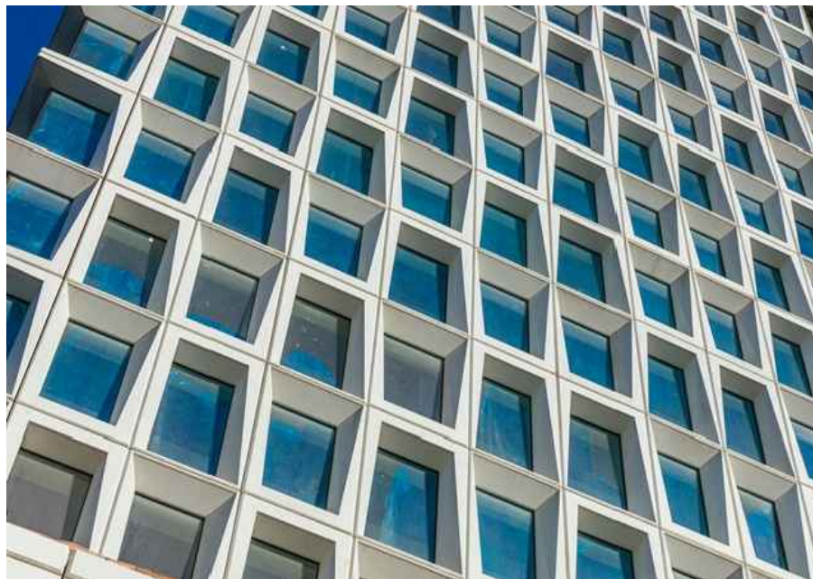
PC-03 PRECAST CONCRETE PANEL - TYPE 2
