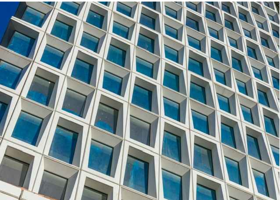
PC-02 PRECAST CONCRETE FRAME
