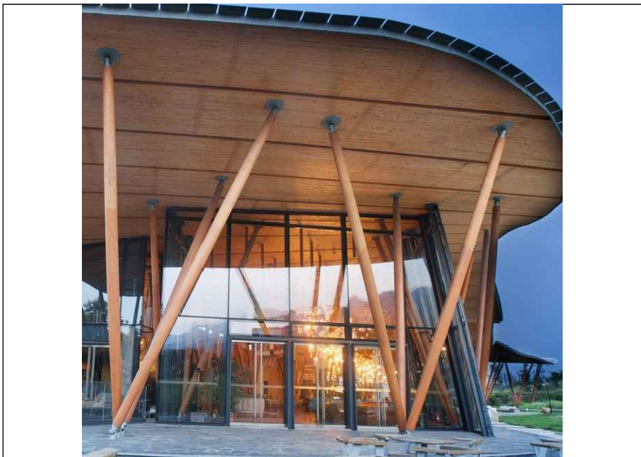
CONC-04 COMPOSITE WOOD CLAD ON CONCRETE COLUMN
