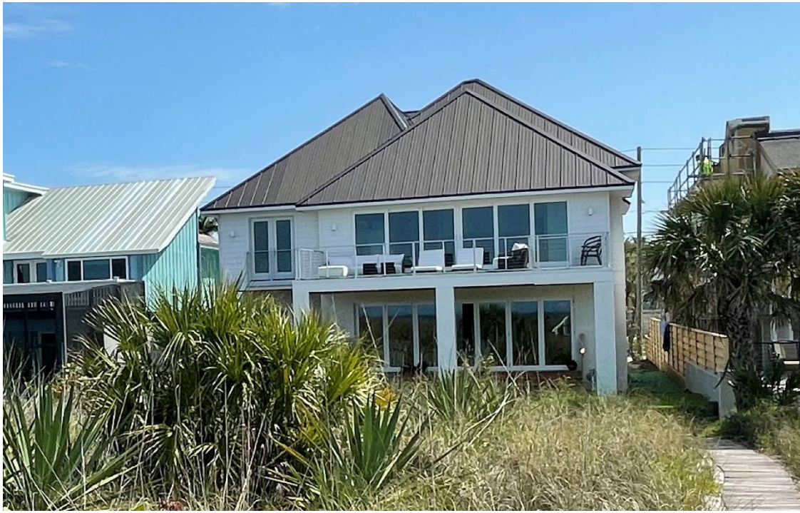
Figure 7: Existing Rear Elevation (staff photo taken 3.13.24)
