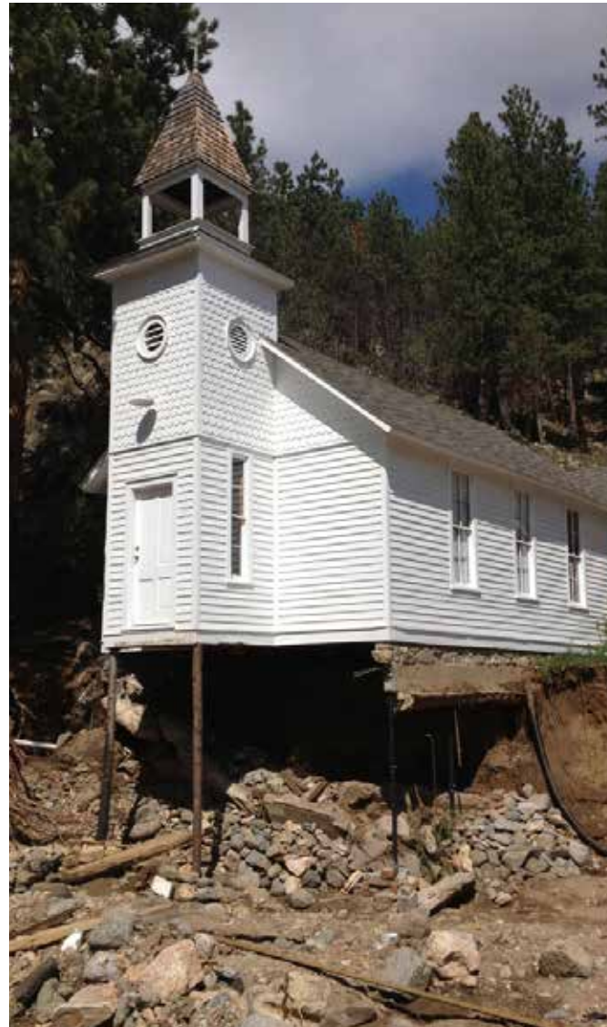
[9] Fast-moving flood waters can undermine a foundation or scour out land around a building. The Little Church of the Pines in Salina, CO, was left structurally compromised after heavy rains caused flooding in the Front Range of the Rocky Mountains in 2013. Photo: Burton Construction burton-construction.com
