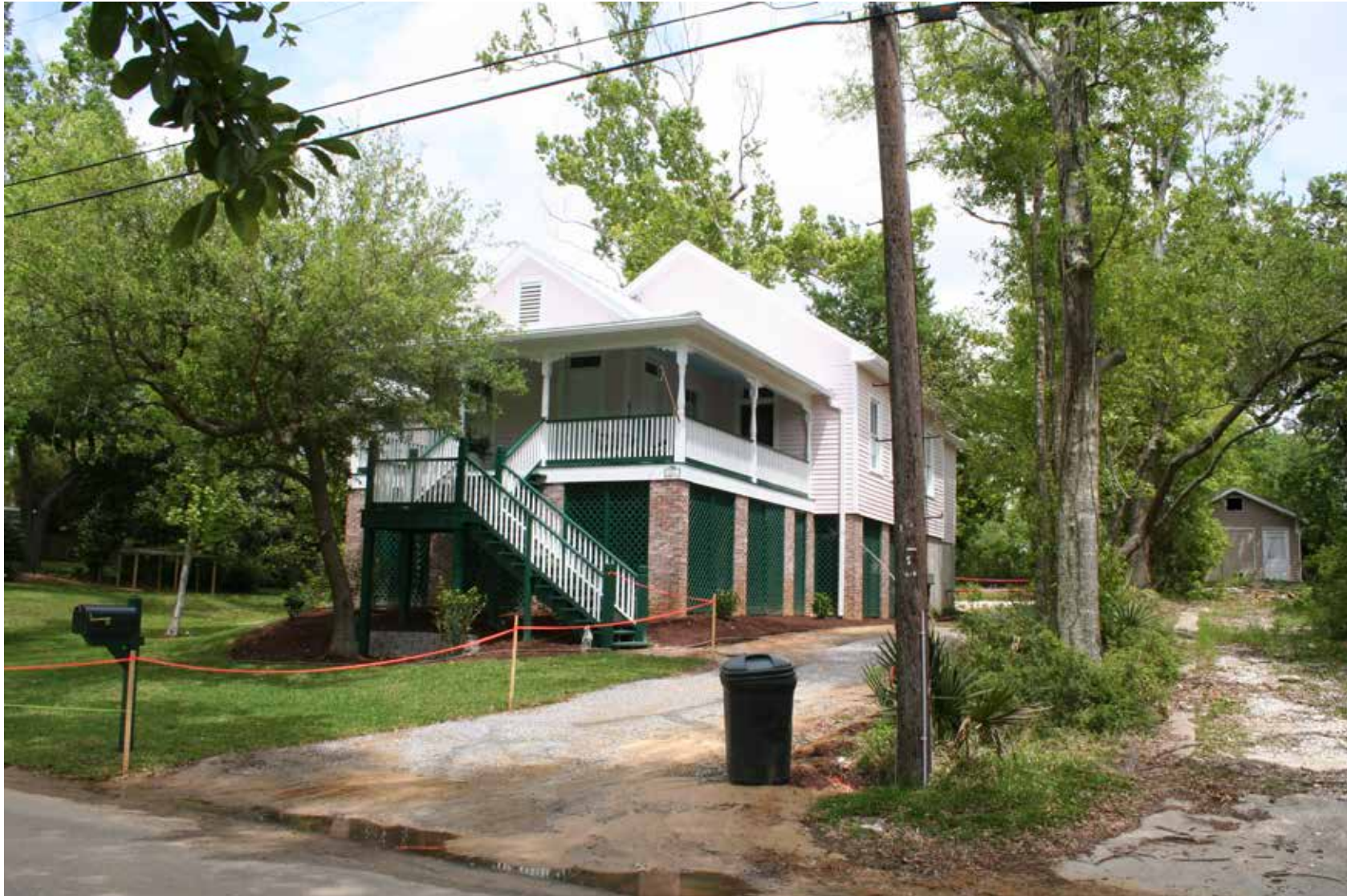
Figure 5: A taller foundation was constructed to elevate the house above the established flood risk level. While the house is higher than it was historically, the change is still in keeping with the historic character of the house, which had been on a tall foundation historically. The change is also consistent with historic regional traditions of adapting buildings to flood events. Additionally, the details of the foundation, with the brick piers and painted lattice, matches features of the historic design. The stairs access the porch in the historic location, but the extended run required by the taller foundation is turned 90 degrees below the landing to allow a surviving tree to remain in front of the house. A small retaining wall behind the tree holds fill that was added around the house to mask some of the change in height. Photo: Mississippi Department of Archives and History, Mississippi Historic Resources Inventory (HRI) Database. http://www.apps.mdah.ms.gov/Public
