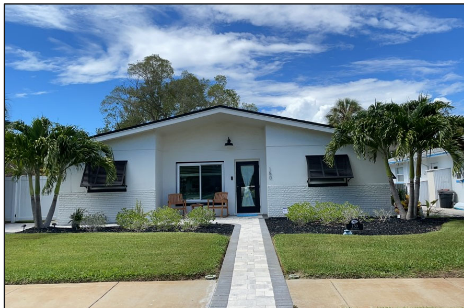
Figure 18. Example of a Contemporary style house, 150 43 rd Ave (8PI16298), within the survey area.
