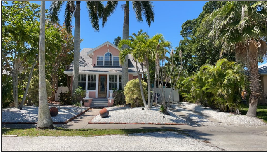
Figure 16. Example of a Bungalow at 3310 E. Maritana Drive (8PI1290) within the survey area.
