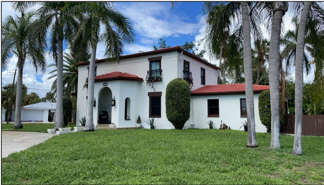
Figure 20. Example of a Mediterranean Revival style residence within the survey area located at 4301 Belle Vista Drive (8PI16300).
