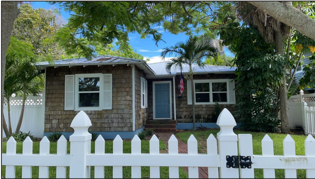
Figure 28. Example of a Frame Vernacular building at 145 43 rd Avenue (8PI16273) within the survey area.
