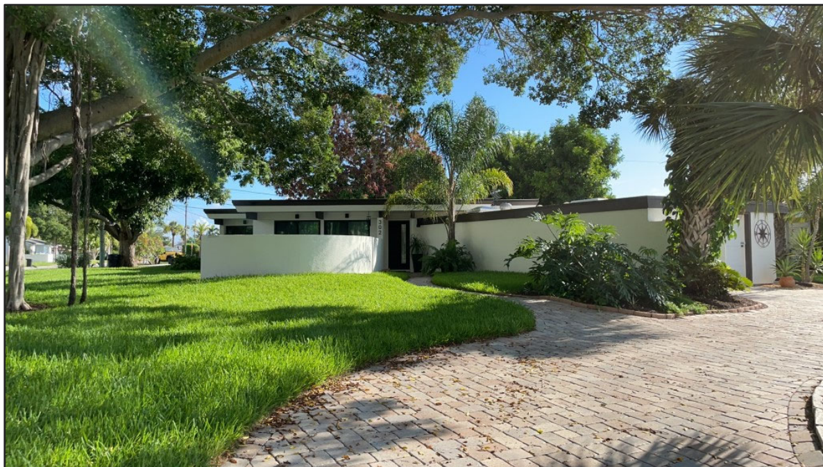
Figure 32. 302 41 st Avenue (8PI16231), south elevation, looking north.
