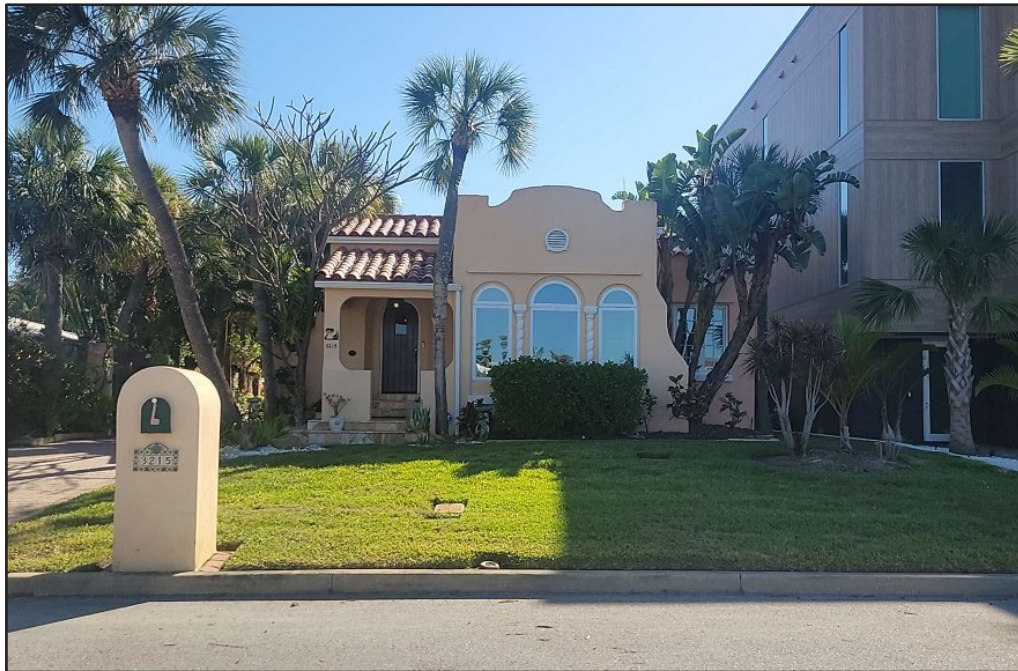
Figure 23. Example of a Mission style house at 3215 W. Maritana Drive (8PI01289), within the survey area.
