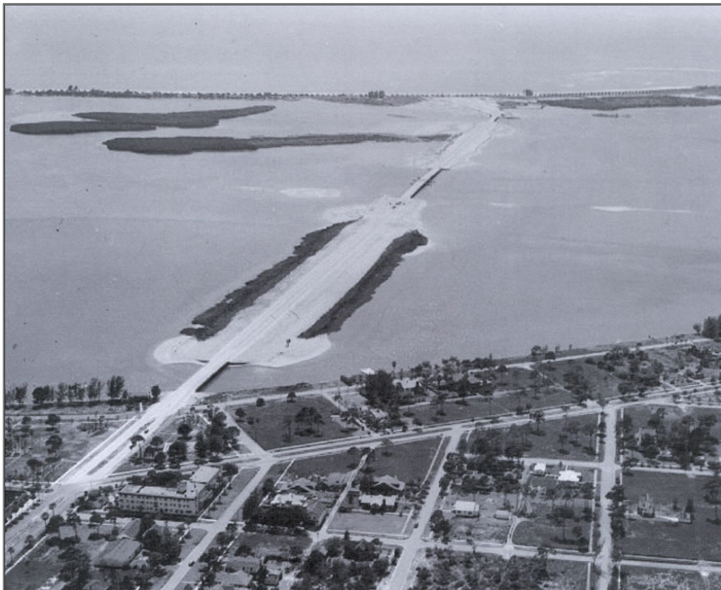
Figure 9. Treasure Island Causeway, ca. 1938, under construction (St. Petersburg Museum of History).
