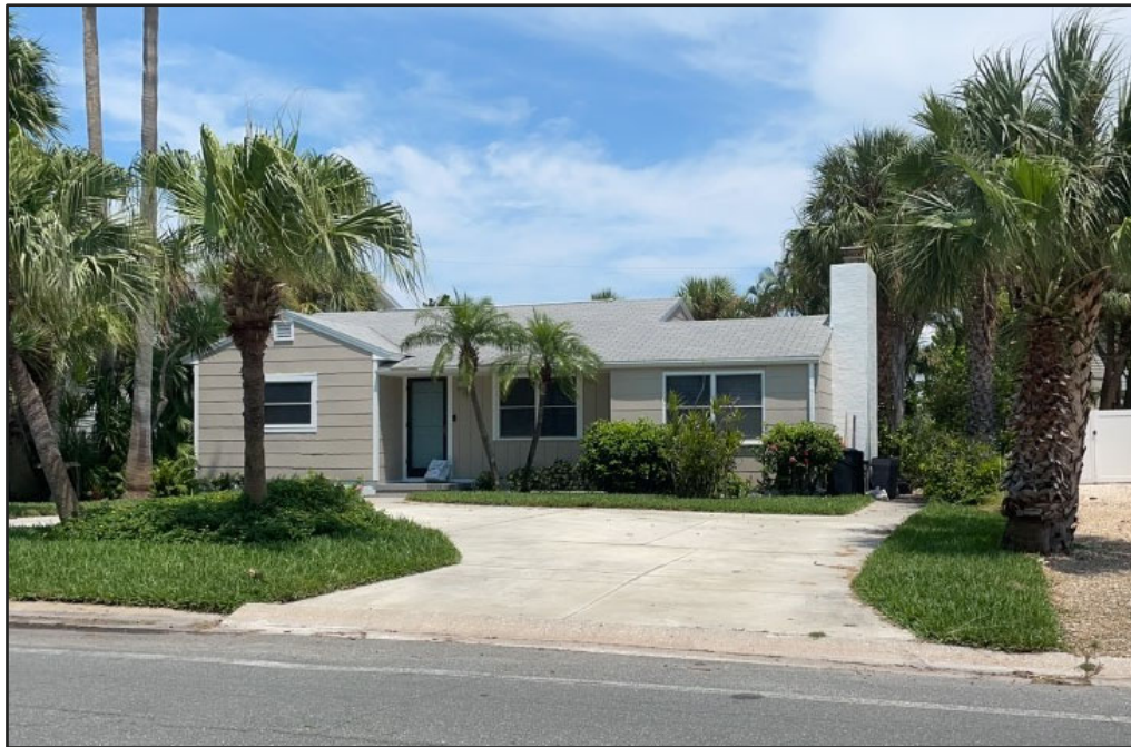
Figure 22. Example of a Minimal Traditional style house at 256 44 th Avenue (8PI16347), within the survey area.
