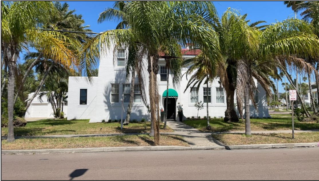
Figure 30. 3401 Casablanca Avenue (8PI01272), west elevation, looking east.
