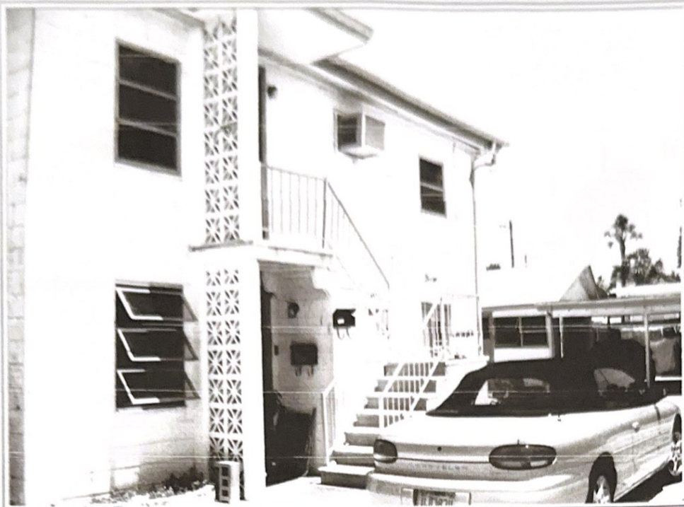
FRONT VIEW OF SUBJECT PROPERTY AT:
