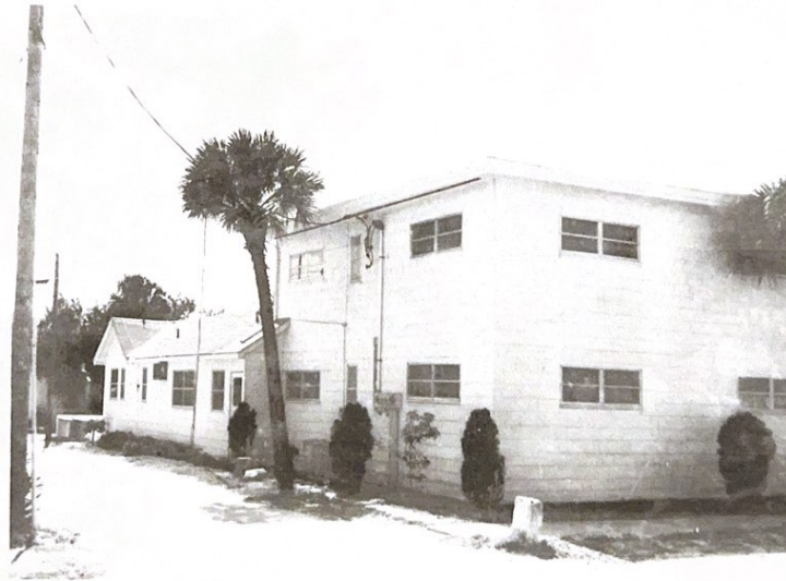
North and Easterly Elevation of Buildings "A" and "B"
