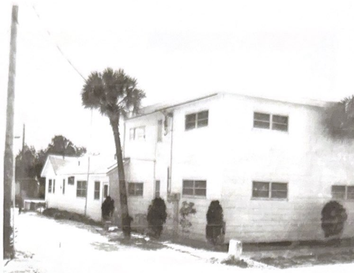
North and Easterly Elevation of Buildings "A" and "B"
