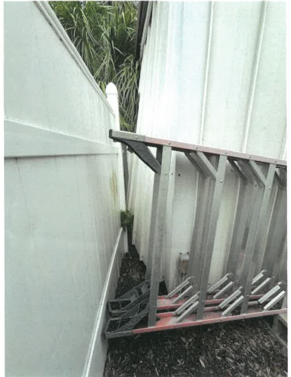
MAINT. SHED - REAR -
