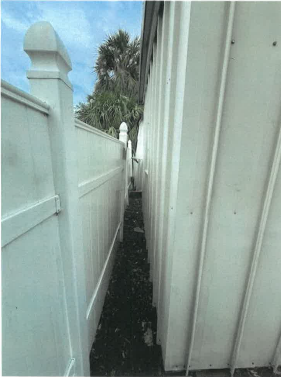
HOBBY SHED - REAR -
