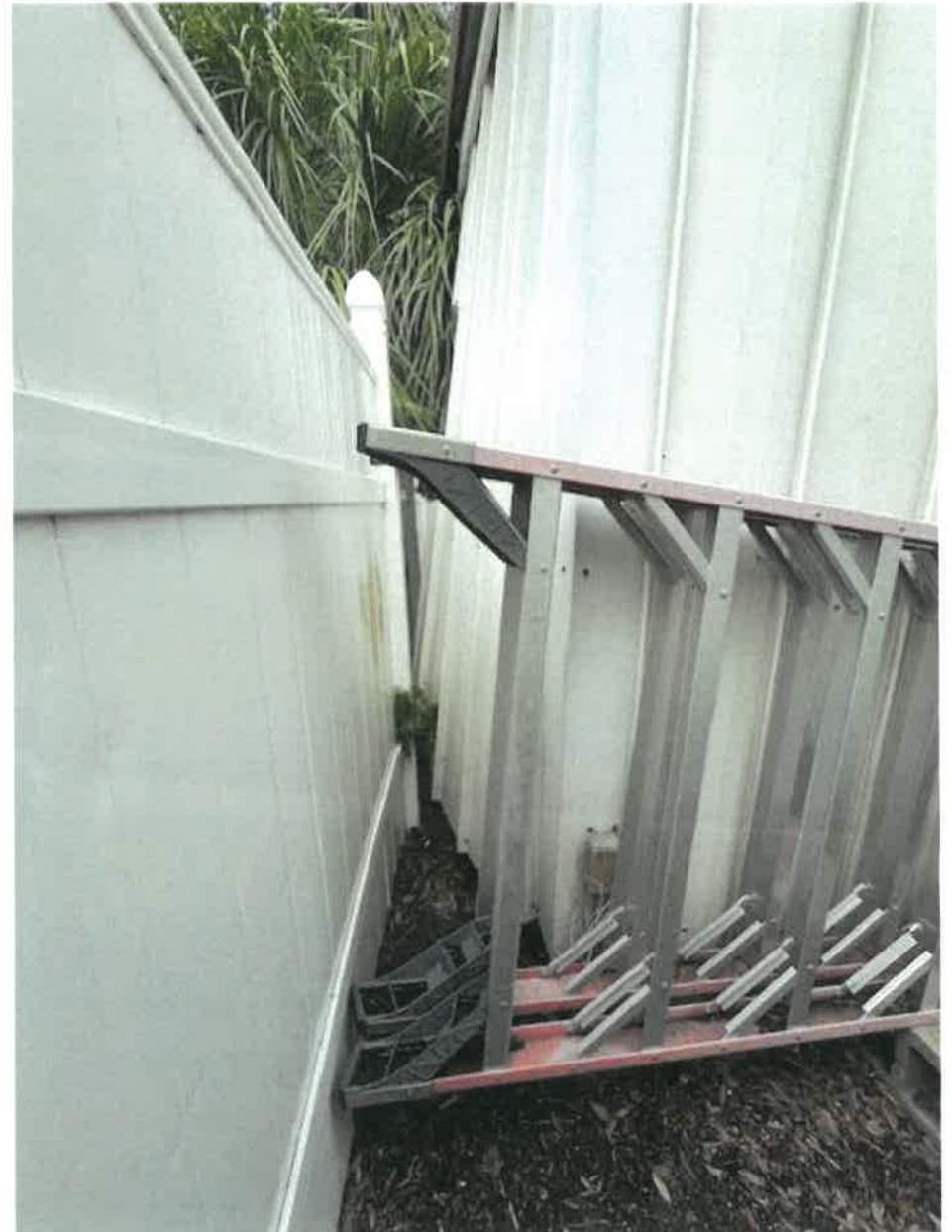
MAINT. SHED - REAR -
