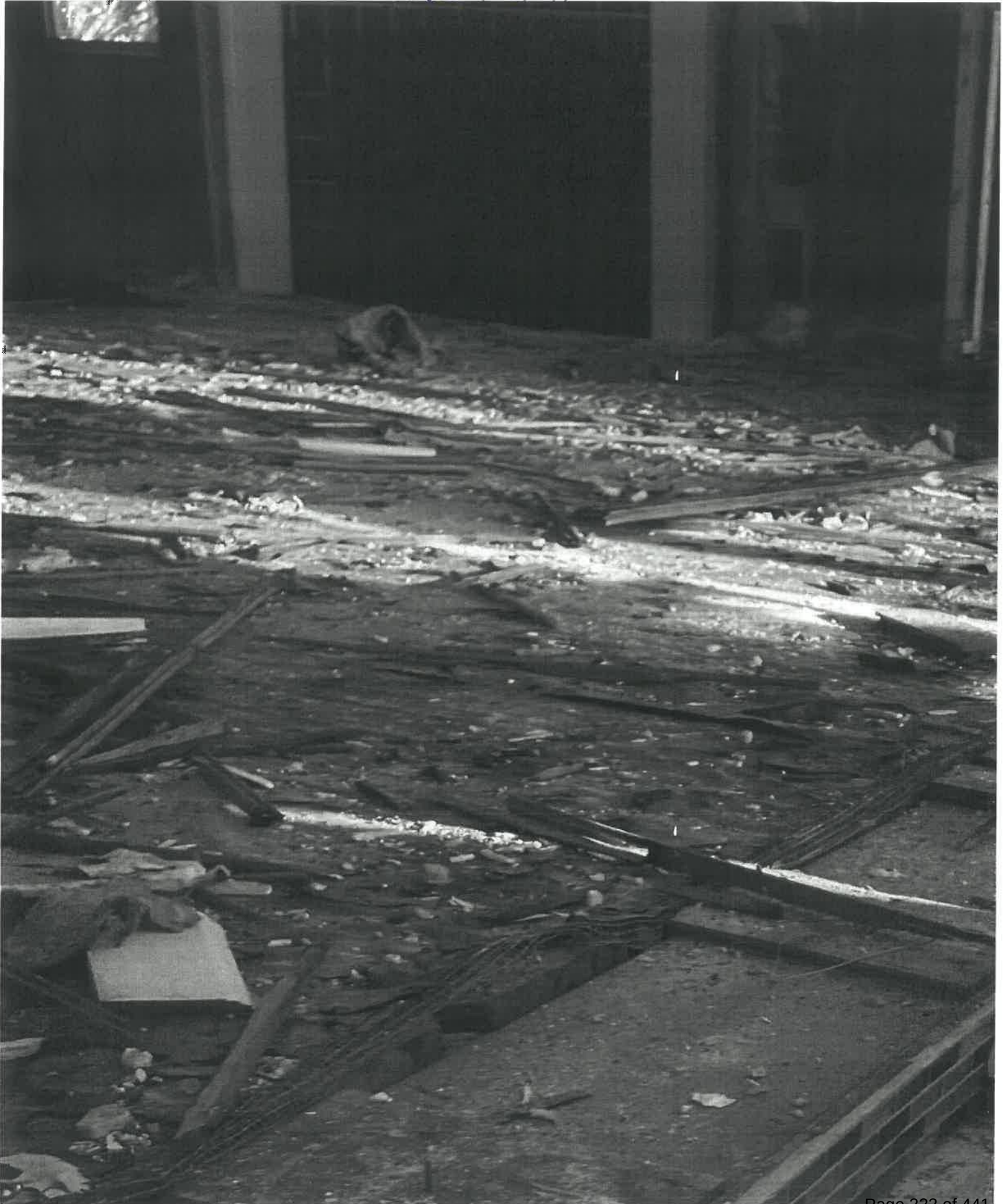
Gutted Interior 1807 Pass A Grille Way Hurricane Helene
