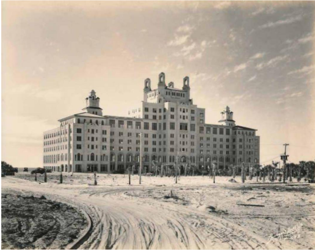
Photo is the Don Cesar Construction from the existing Vantage Point of the DeBazan Ave, and essentially the 5 Villas.
