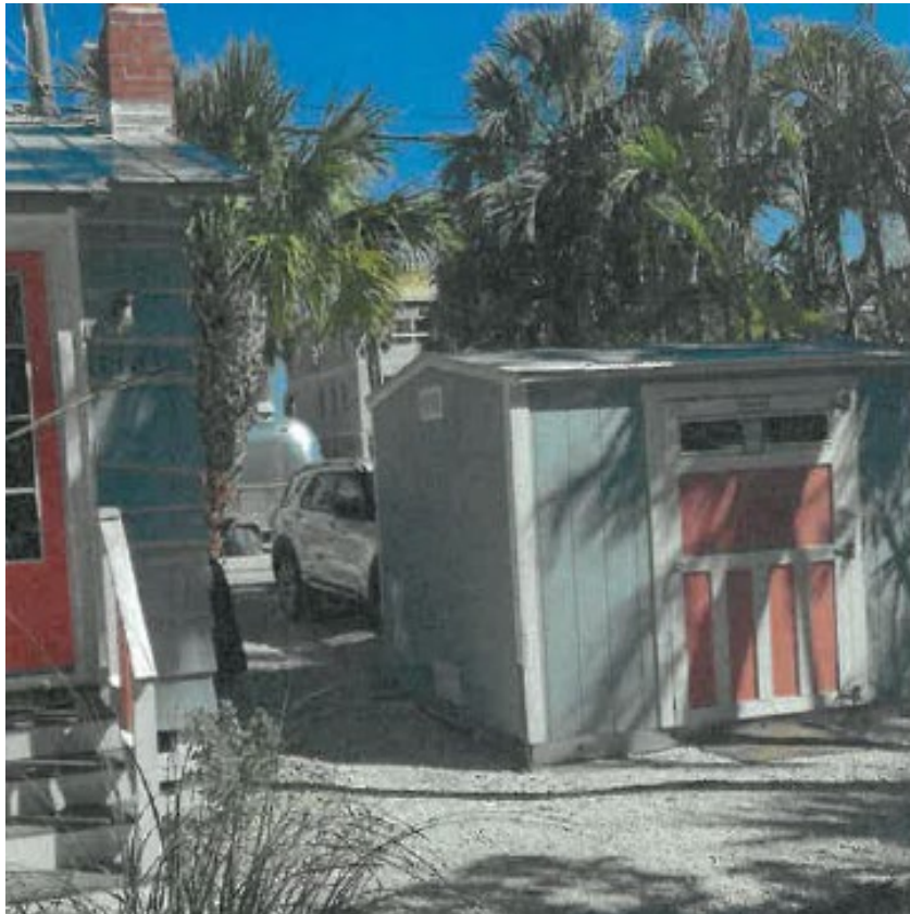
Recently Installed Storage Building
