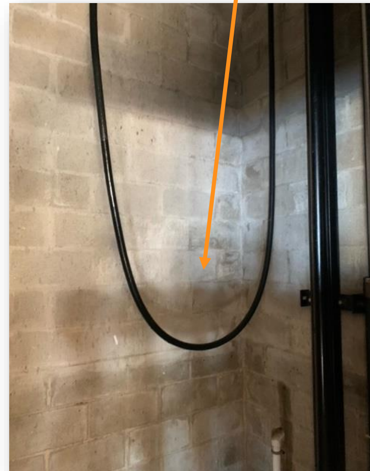
From route technician visiting jobsite right after hurricane.
