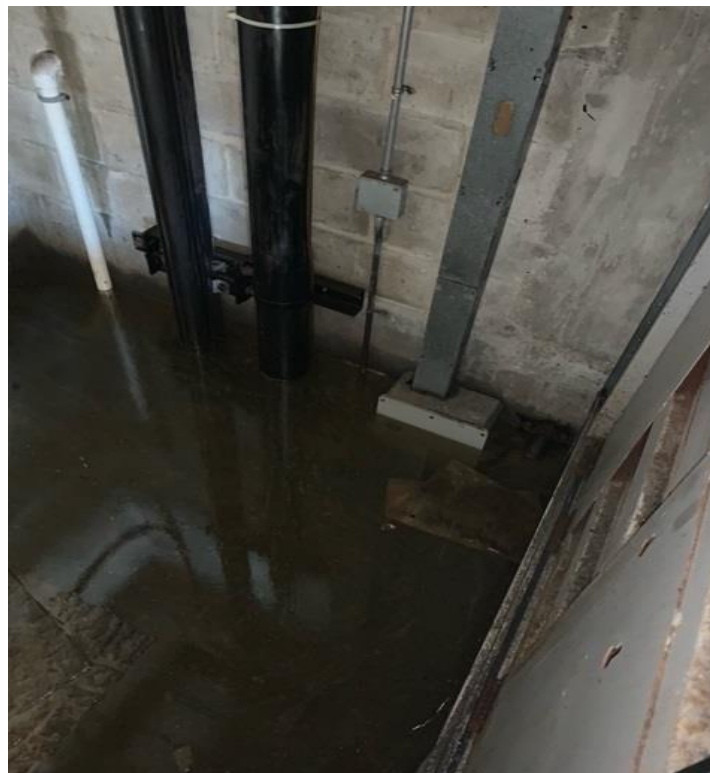
Storm survey. Water in pit. Pit stop switch, travel cable, shaft wiring, and rust remediation. Left unit down.
