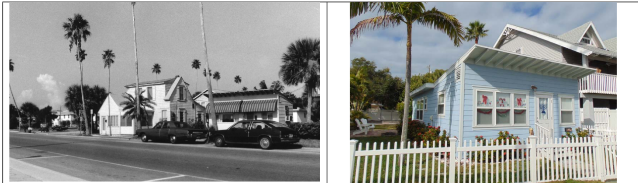
Above, left: The structure, photographed in 1989, showing its original board siding and fabric awnings over the front entrance.
