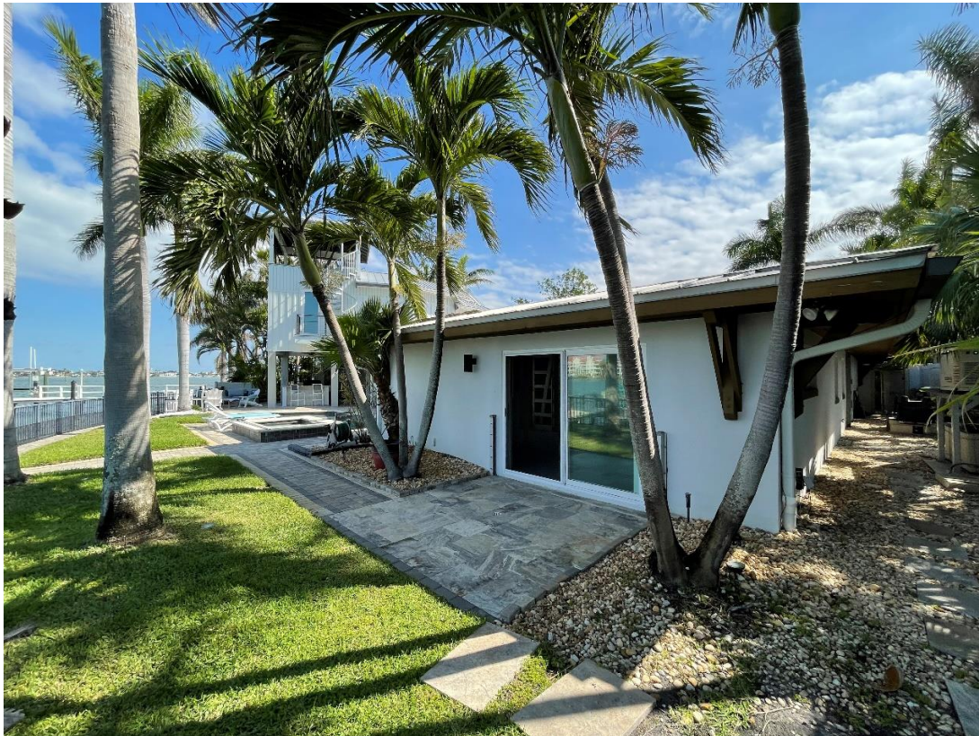
View from the south looking north
