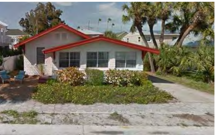
Figure 4: Home featuring enclosed front porch, shingled siding, narrow side drive aisle to enclosed 2-story guest cottage
