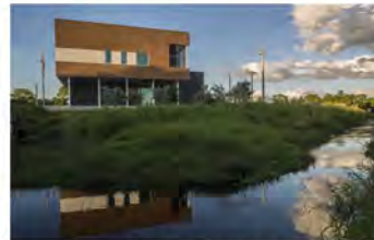
SARASOTA COUNTY FIRE STATION #14, SARASOTA, FL
