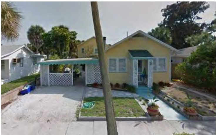
Figure 3: Home featuring carport addition
