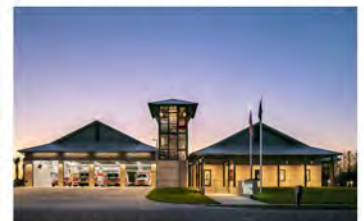
SARASOTA COUNTY FIRE STATION #8, SARASOTA, FL
