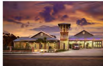
SARASOTA COUNTY FIRE STATION #1, SARASOTA, FL
