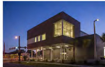
SARASOTA COUNTY FIRE STATION #12, SARASOTA, FL
