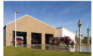
BOKEELIA FIRE STATION #3 PINE ISLAND, FL
