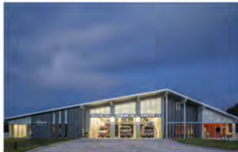
SARASOTA COUNTY FIRE STATION #16, SARASOTA, FL
