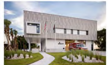
SARASOTA COUNTY FIRE STATION #13, SIESTA KEY, FL
