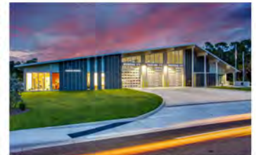
SARASOTA COUNTY FIRE STATION #17, SARASOTA, FL
