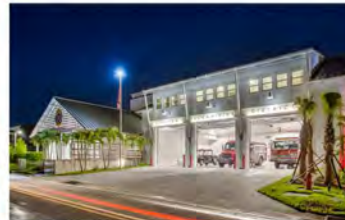
CAPTIVA ISLAND FIRE STATION CAPTIVA, FL
