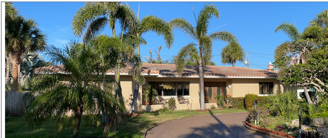
The structure photographed in 2024 for its Florida Master Site File. The residence has been effectively unaltered since the 1990s, with no noted permits on record. Additions were made to the rear side and rear secondary front of the structure in the 1990s, which did not meaningfully alter the view of the structure from its frontage.
