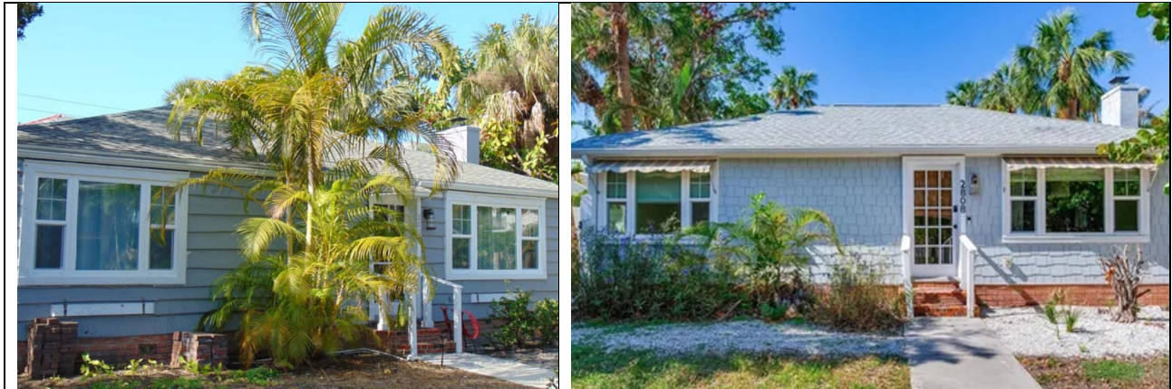
Above, left: The front residence photographed in 2015 for the City's historic resources survey. Above, right: The residence photographed by the owner in 2025, showing the cedar shake replacement siding.
