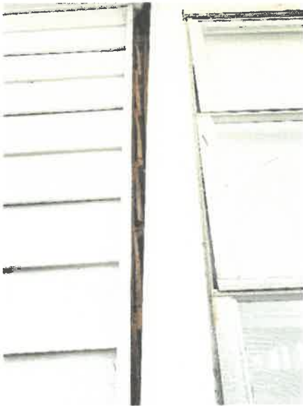
Observation 11: Opening in wall
