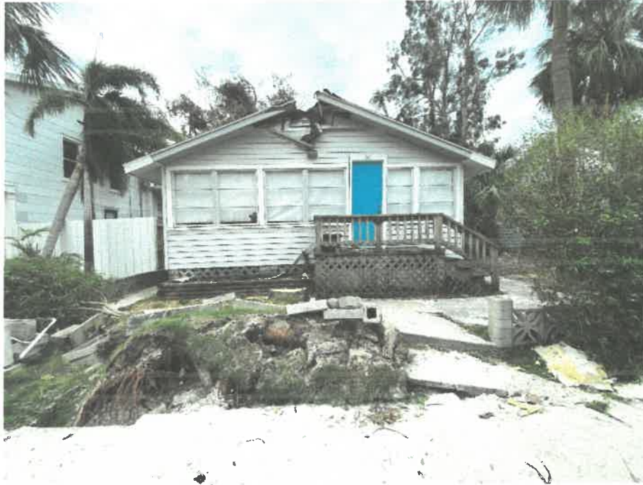
Photo 2: Front View of Building. (North)
