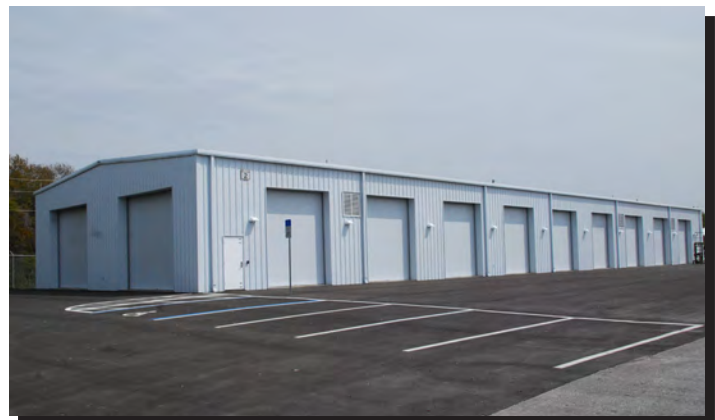
Pinellas County Public Works Vehicle Storage Facility
