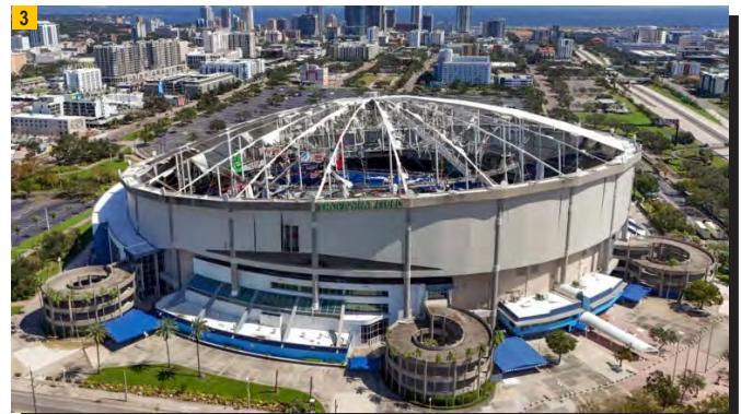
Tropicana Field Repairs & Roof Replacement
