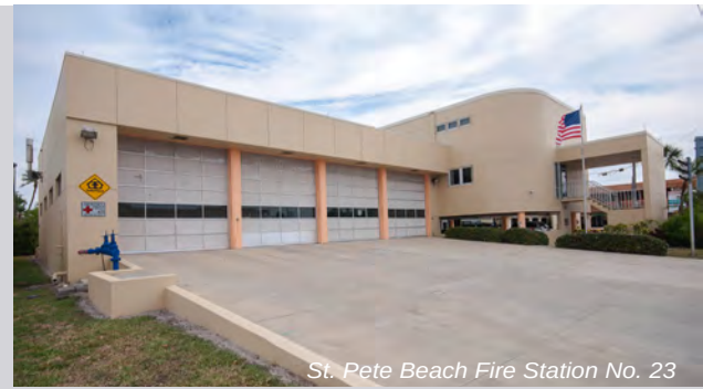
St. Pete Beach Fire Station No. 23
