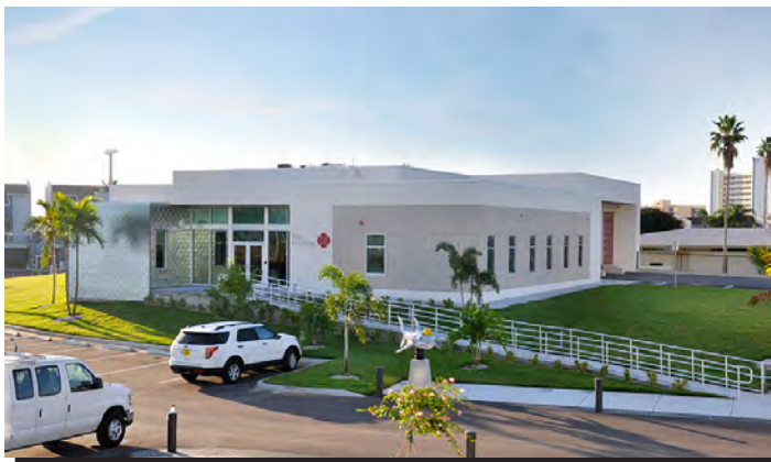
Madeira Beach Fire Station
