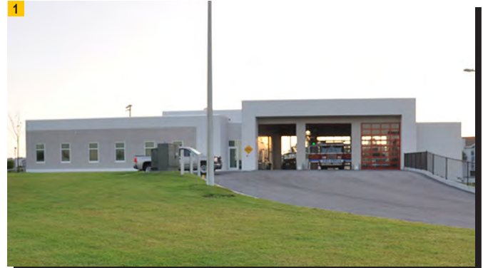
Madeira Beach Fire Station
